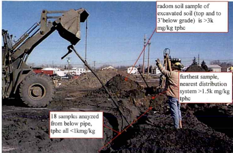
Jan. 15, gas pipe excavation / removal from the fuel distribution/railroad track area sample results show a clean excavation and approx. 50 ft. of the pipe-run has been backfilled.
