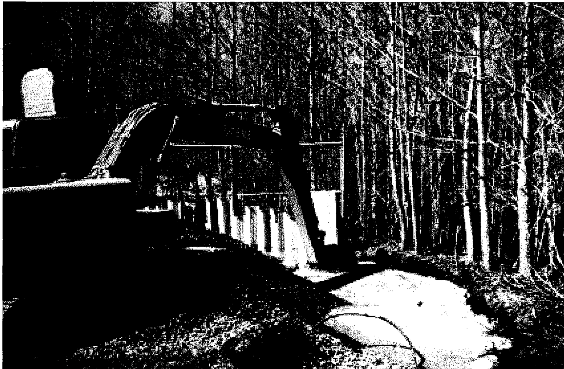
Vinyl sheeting was driven along the north and east end of the excavation to prevent creek erosion and the migration of contaminants.
