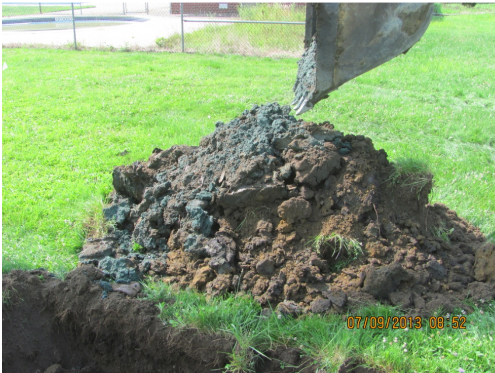
6. IMG006 Test Pit FFSGC-E.
