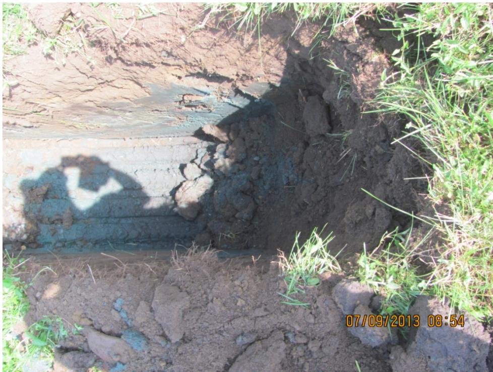
9. IMG009 Test Pit FFSGC-E.
