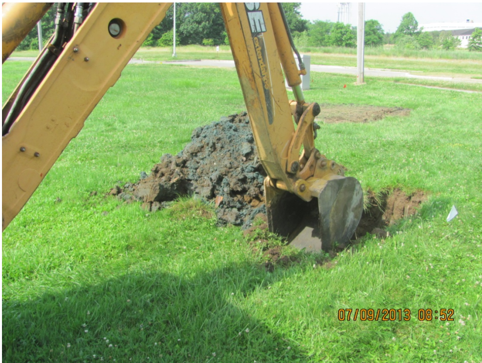
8. IMG008 Test Pit FFSGC-E.
