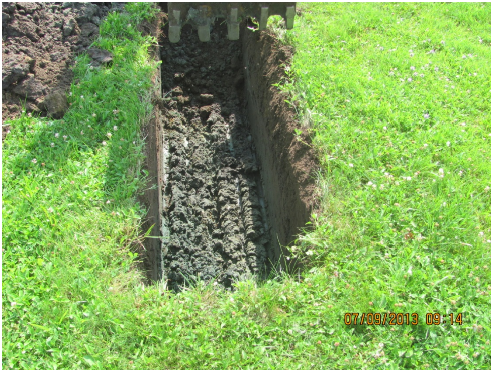
11. IMG011 Test Pit FFSGC-D. Field notes indicate “Brown-green glauconitic sand and clay with dark black-brown natural clay at 4.5 ft, no odor or debris.”
