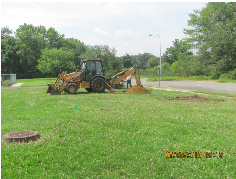
17. IMG017 Excavating Test Pit SUST-C; Test Pit SUST-B has been backfilled to the right.
