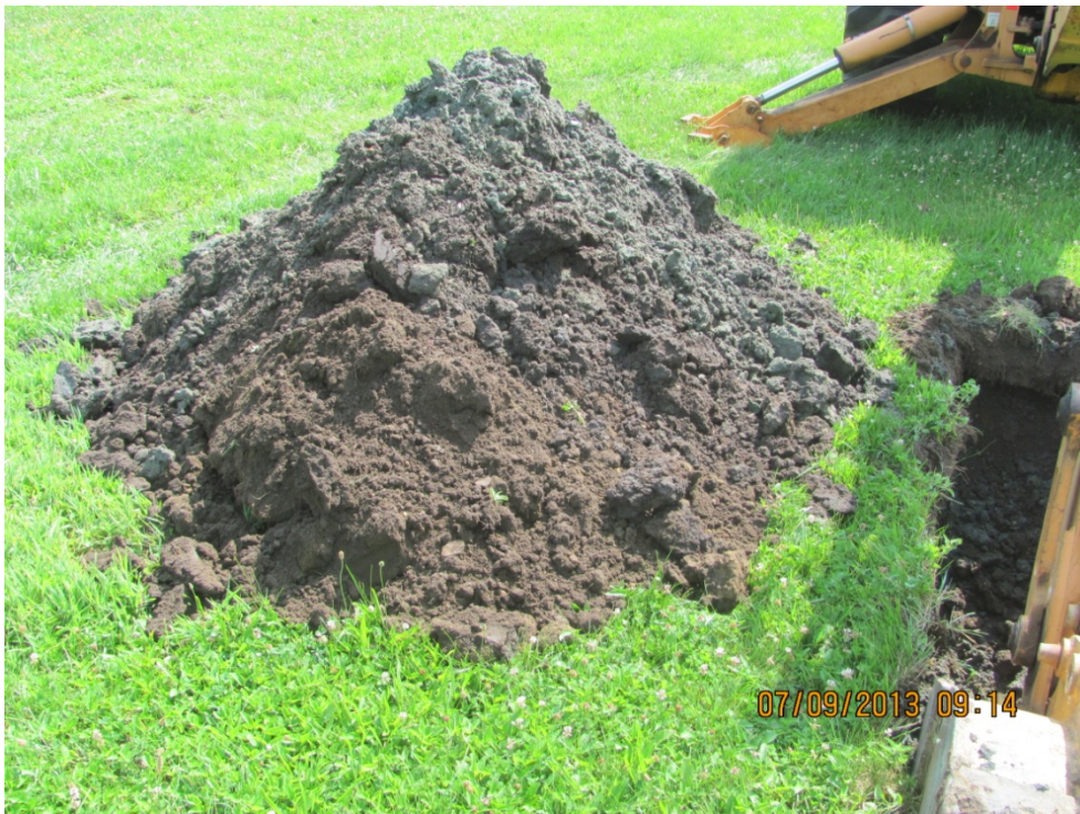
12. IMG012 Test Pit FFSGC-D.
