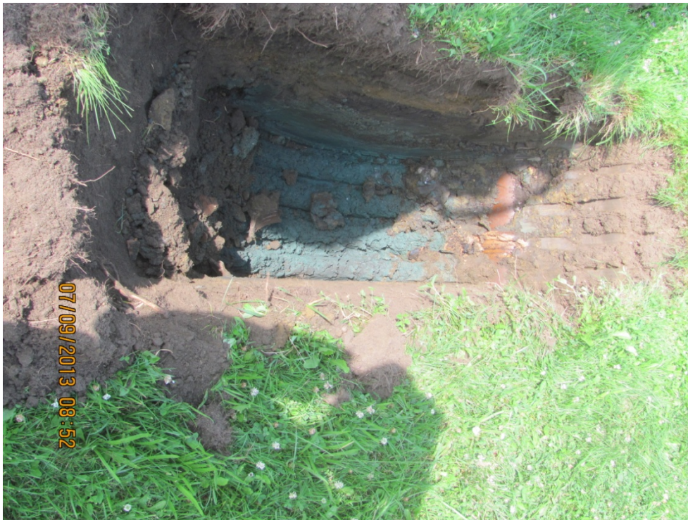
7. IMG007 Test Pit FFSGC-E. Buried terracotta pipe shown on right.
