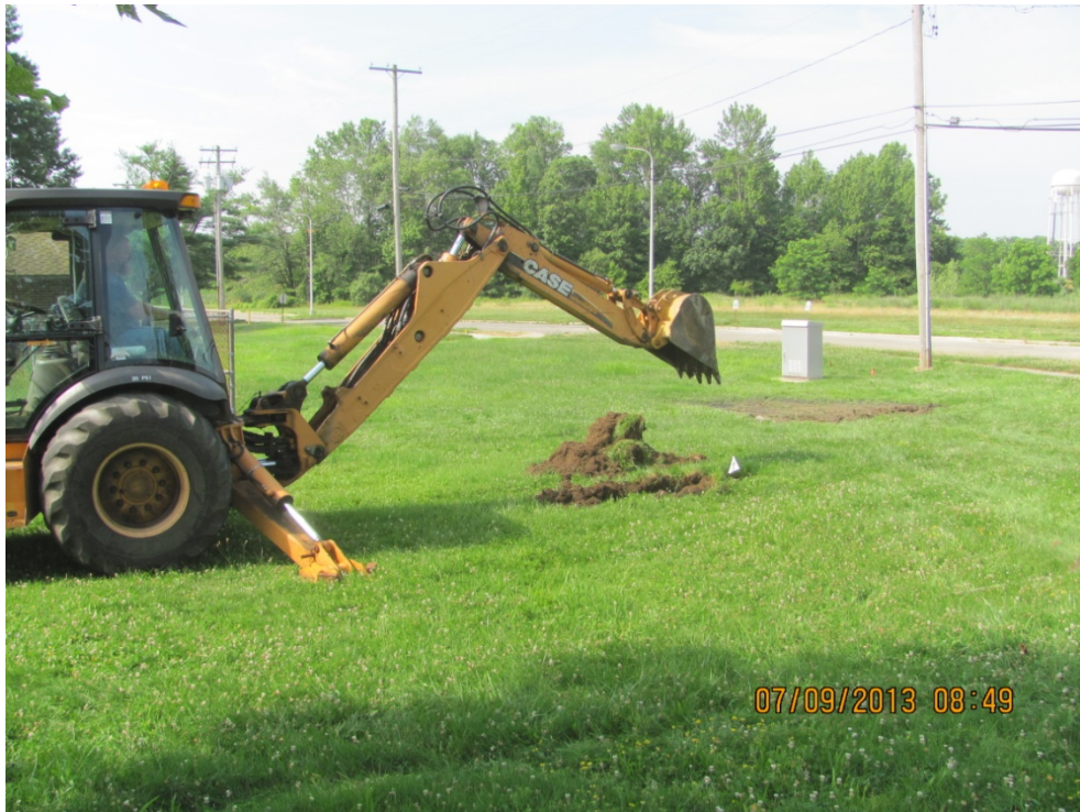
4. IMG004 Test Pit FFSGC-E during excavation. View facing southwest.
