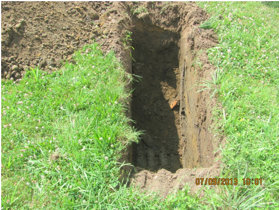
16. IMG016 Test Pit SUST-B.
