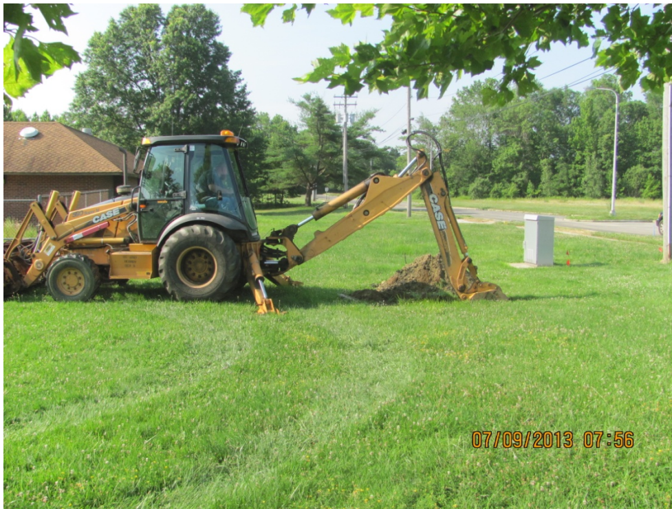
1. IMG001 Test Pit FFSGC-C during excavation. View facing south; Building 2569 on the left.
