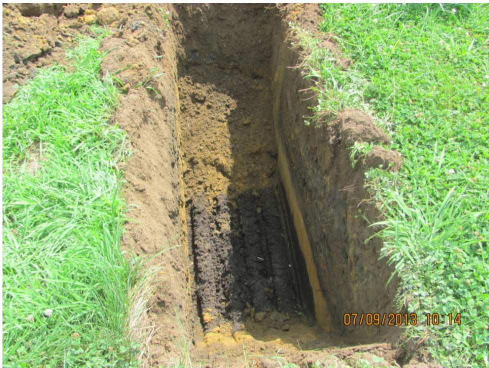
18. IMG018 Test Pit SUST-C. Field notes indicate "Brown medium sand with petroleum odor at 4.5 feet, and black-gray stained soil." Soil sampled at 5.0 to 5.5 feet.
