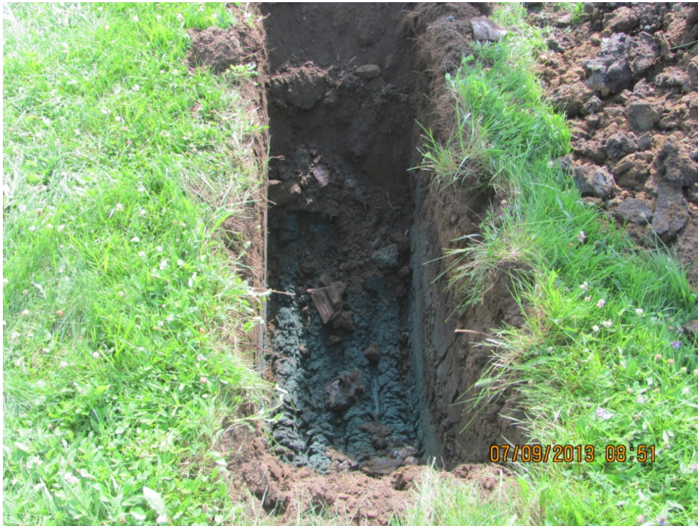
5. IMG005 Test Pit FFSGC-E. Field notes indicated "Terracotta pipe, brown-green glauconitic sand with clay, burnt wood pieces."
