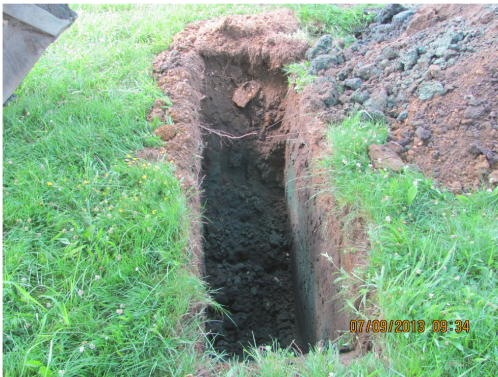
14. IMG014 Test Pit FFSGC-B. Field notes indicate “pea gravel mixed with brown-orange fill sand, glauconitic clay at 4.5 feet.”
