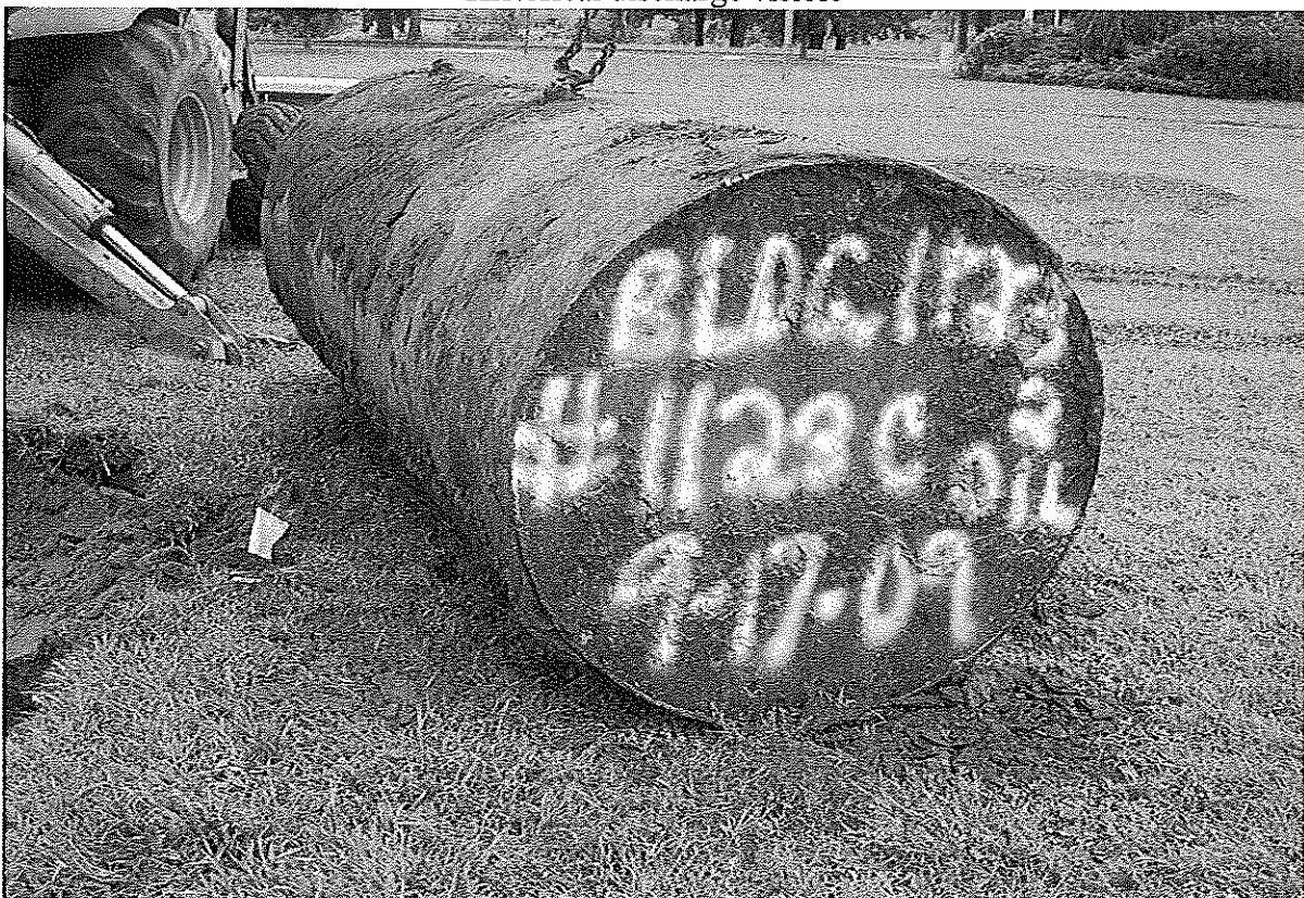
Second UHOT removed from Bldg. 1123
