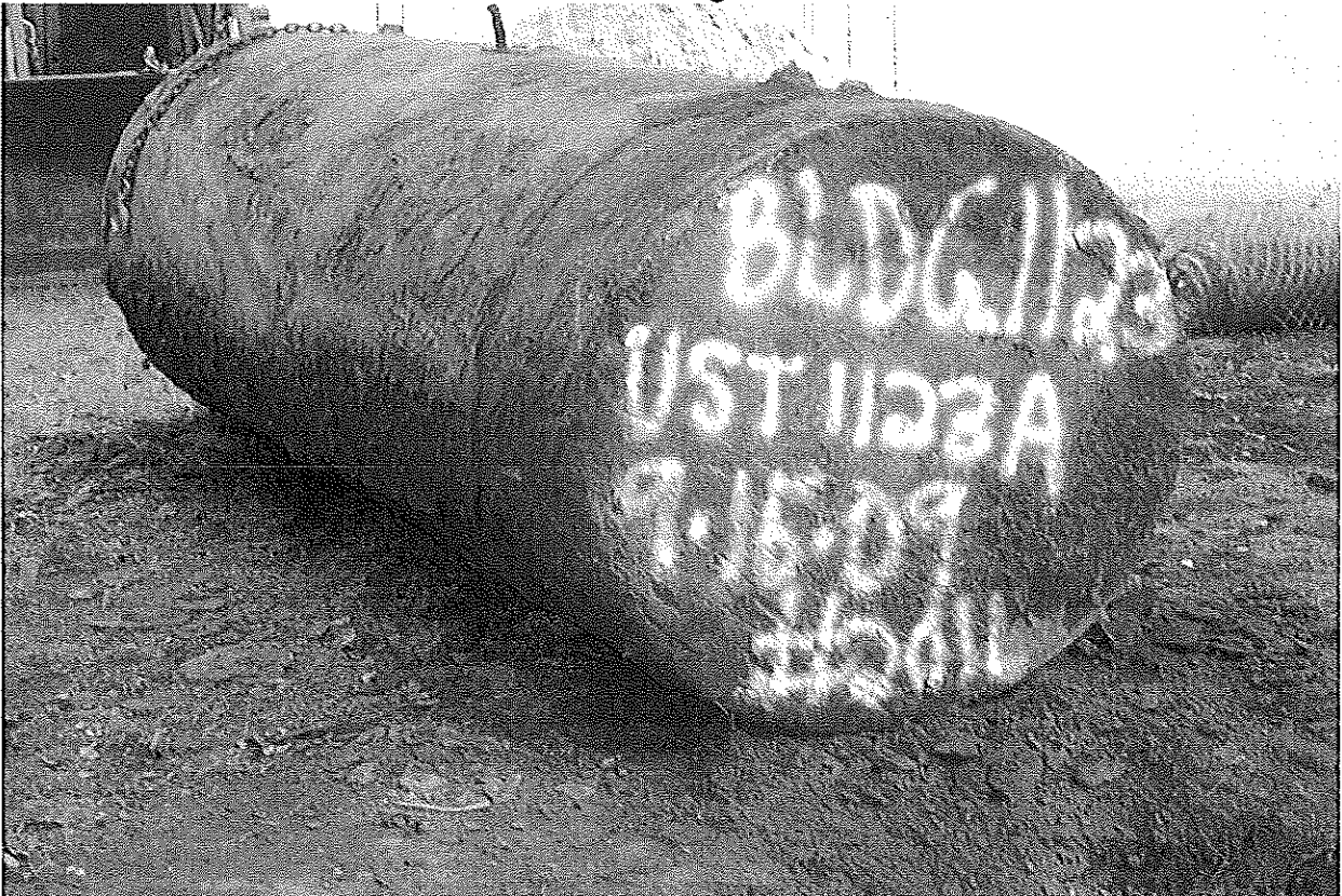
UHOT removed from excavation
