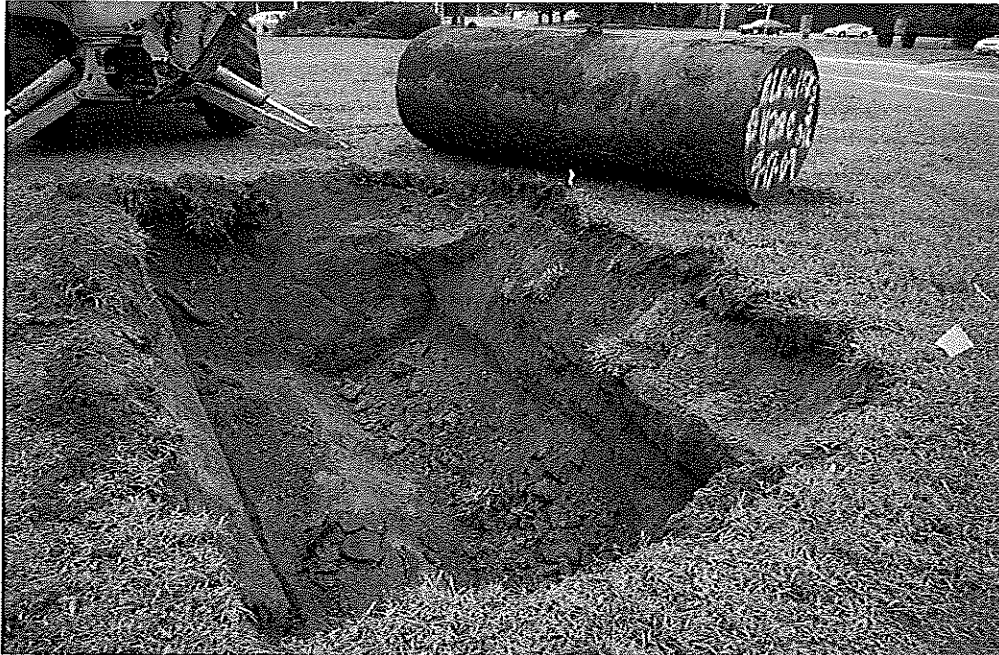
Excavation of second UHOT, note staining in bottom left of photo
