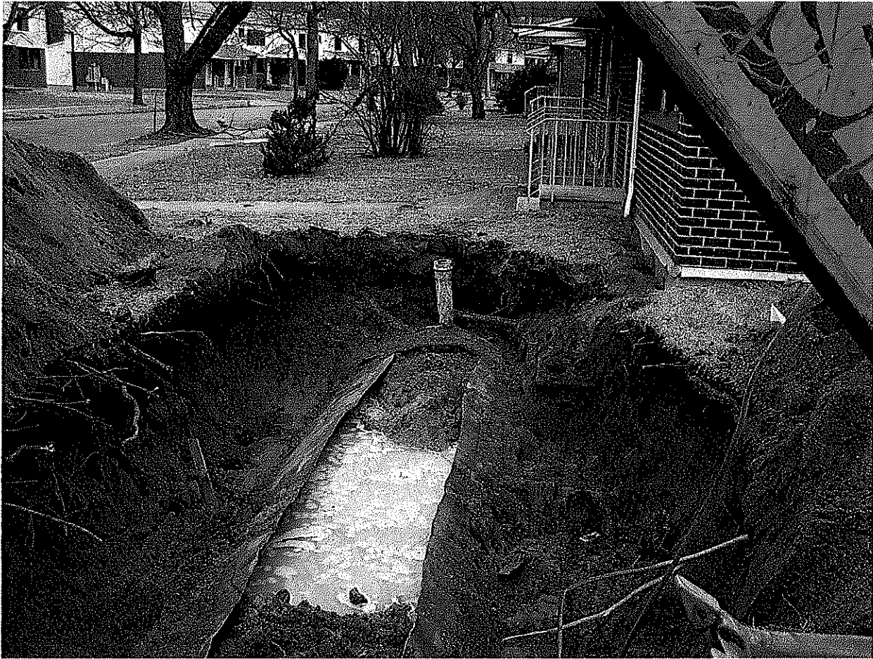
Top of sand filled tank exposed
