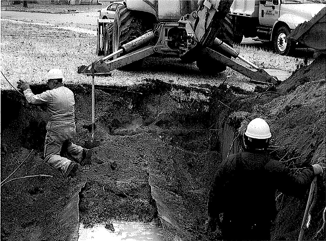
PULLING LINES BACK TO ALLOW FOR ACCESS TO TANK
