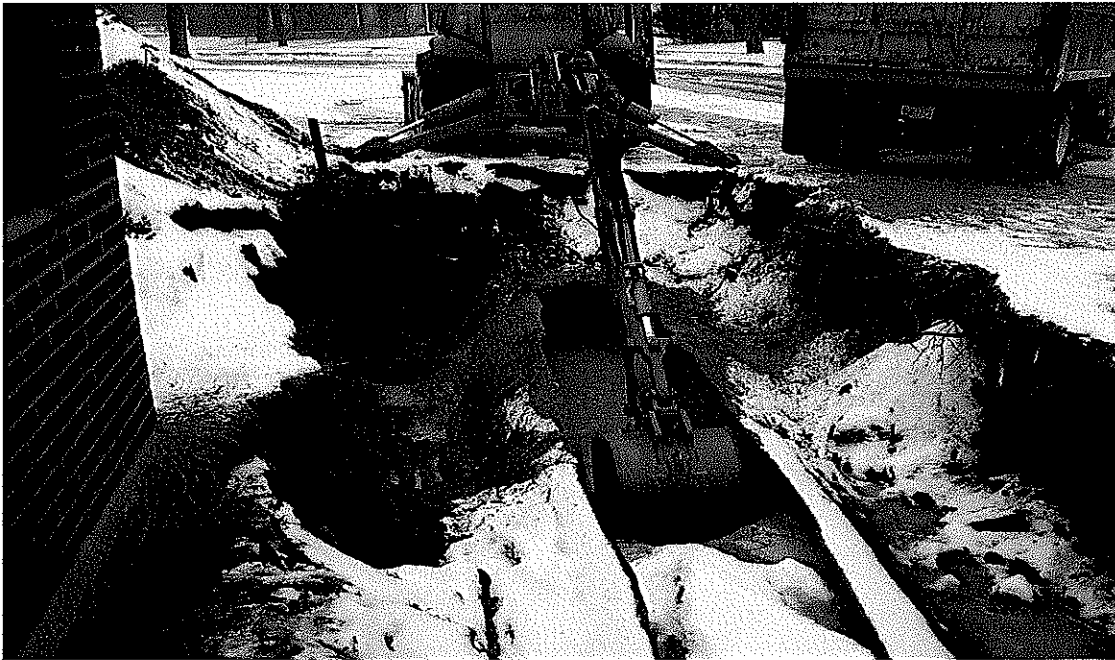
REMOVING SAND FROM TANK
