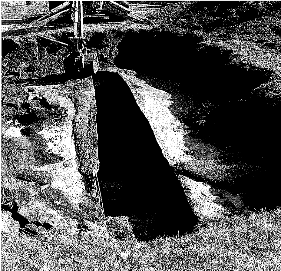
Tank emptied of the sand contents
