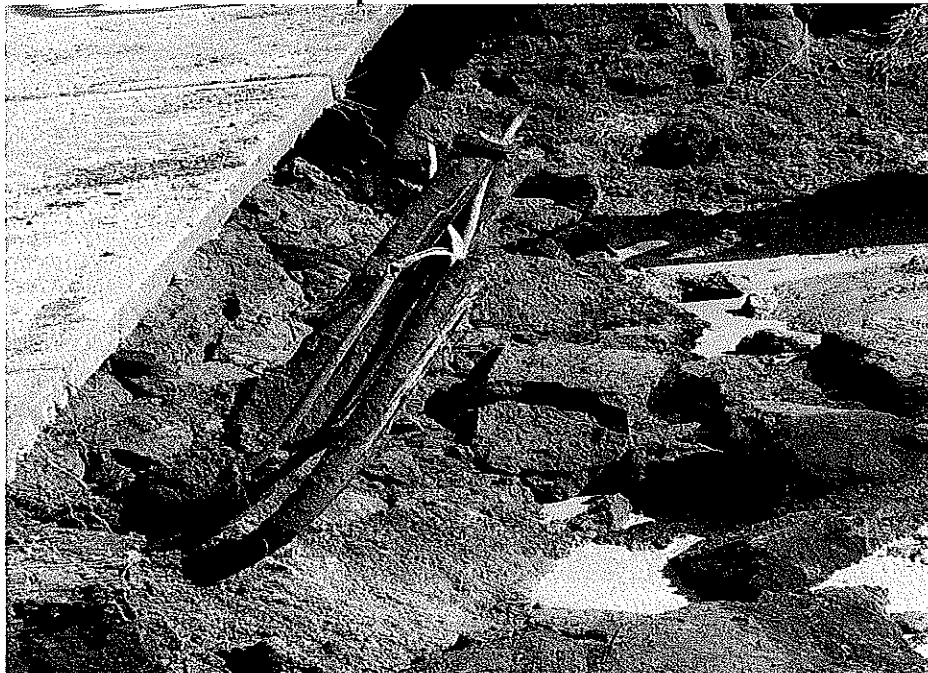
CUT UTILITY LINES IN THE EXCAVATION
