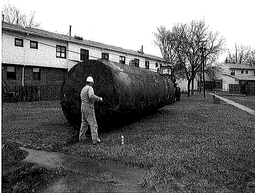
TANK REMOVED FROM GROUND
