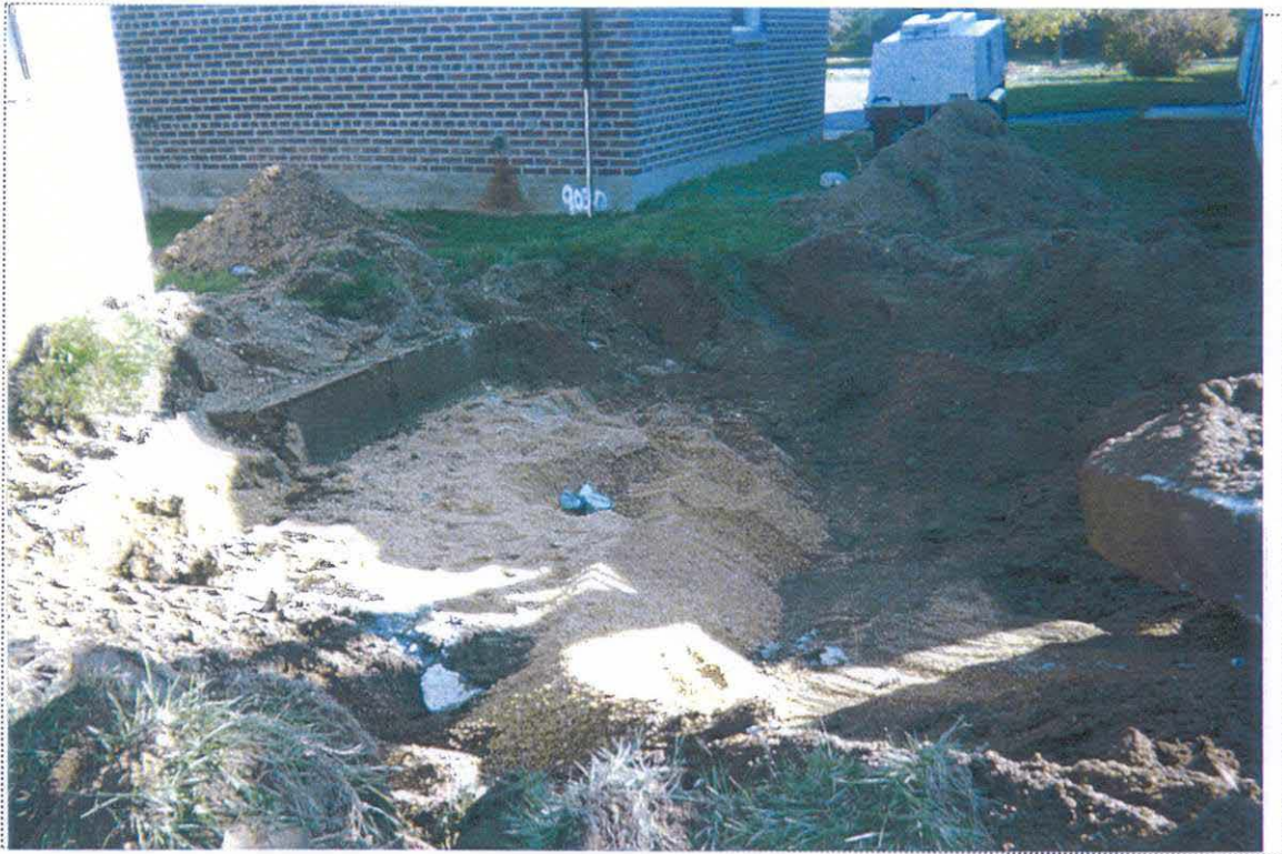
PHOTO 1: View of excavation activities commencing at the UST-9030 location (looking south/southeast).
