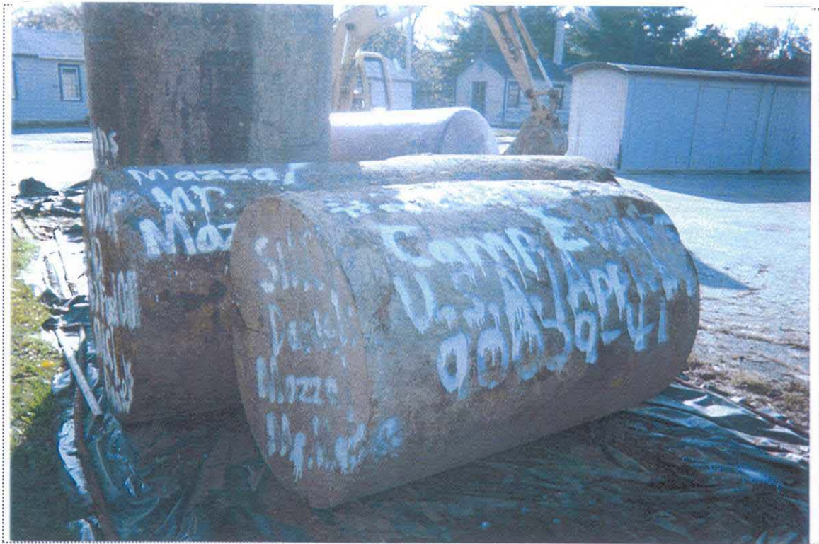
PHOTO 3: View of UST-9057(A) staged on the west side of Building 9061 awaiting disposal and labeled with all required information.
