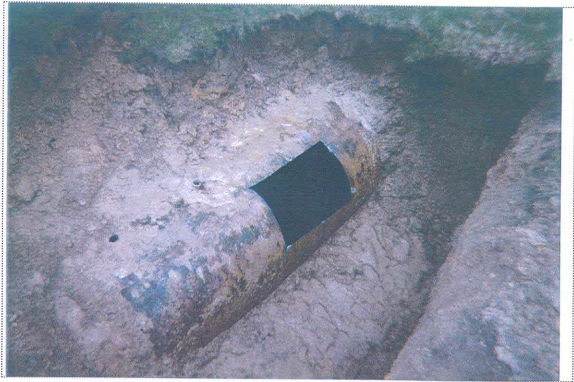
PHOTO 1: View of UST-9053 after completion of cleaning activities (looking southwest).
