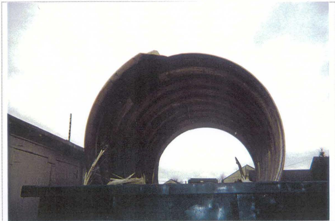
PHOTO 4: View of a section of UST-9064 in the rolloff container waiting to be crushed prior to ultimate disposal (looking north).
