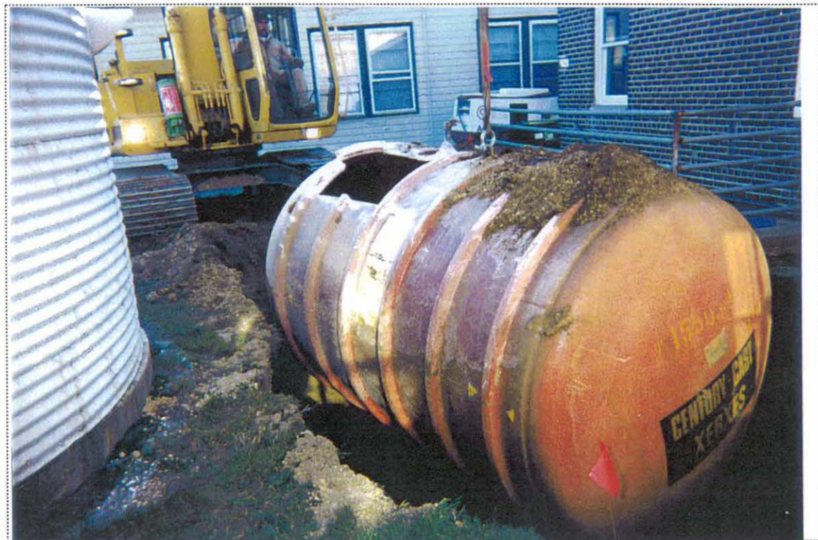
PHOTO 2: View of the UST-9028(A) being removed from the ground (looking west/northwest).
