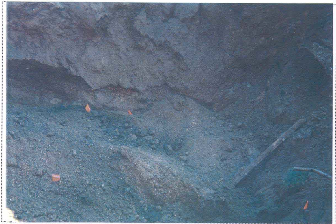
PHOTO 4: View of the sampling locations in the UST-9035 excavation (looking southwest).
