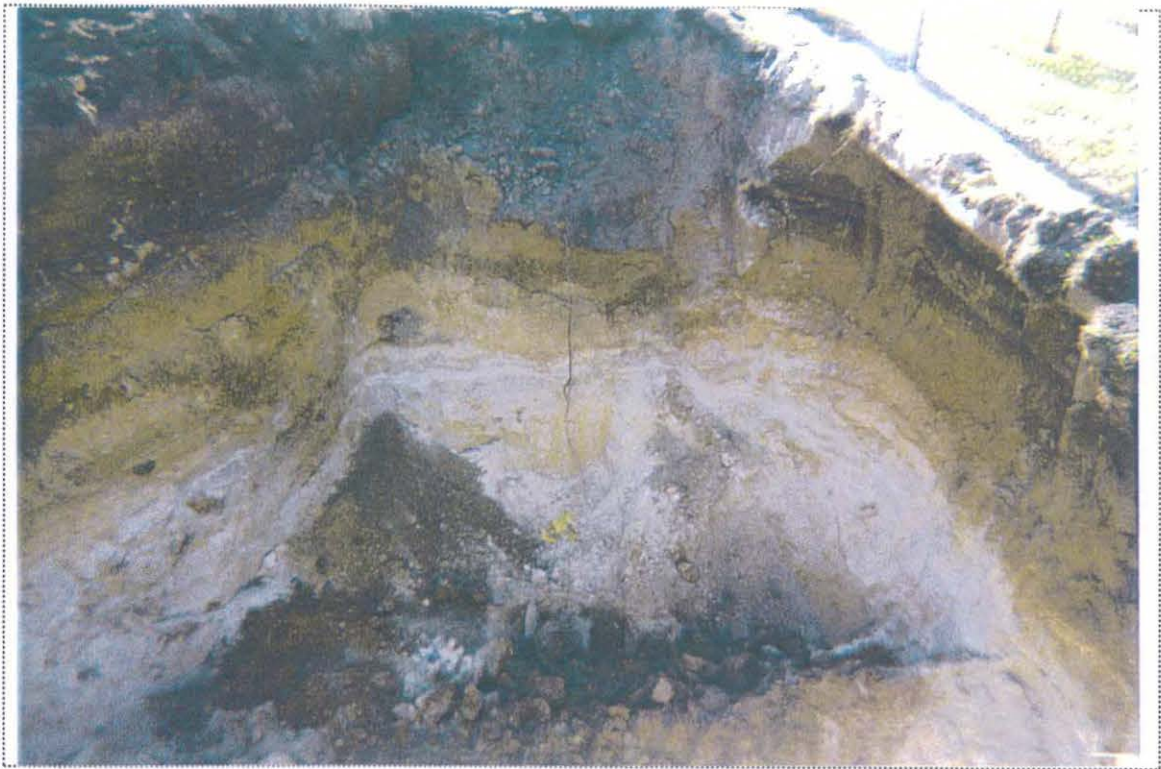
PHOTO 3: View of the remedial excavation at the former UST-9031 location (looking west).
