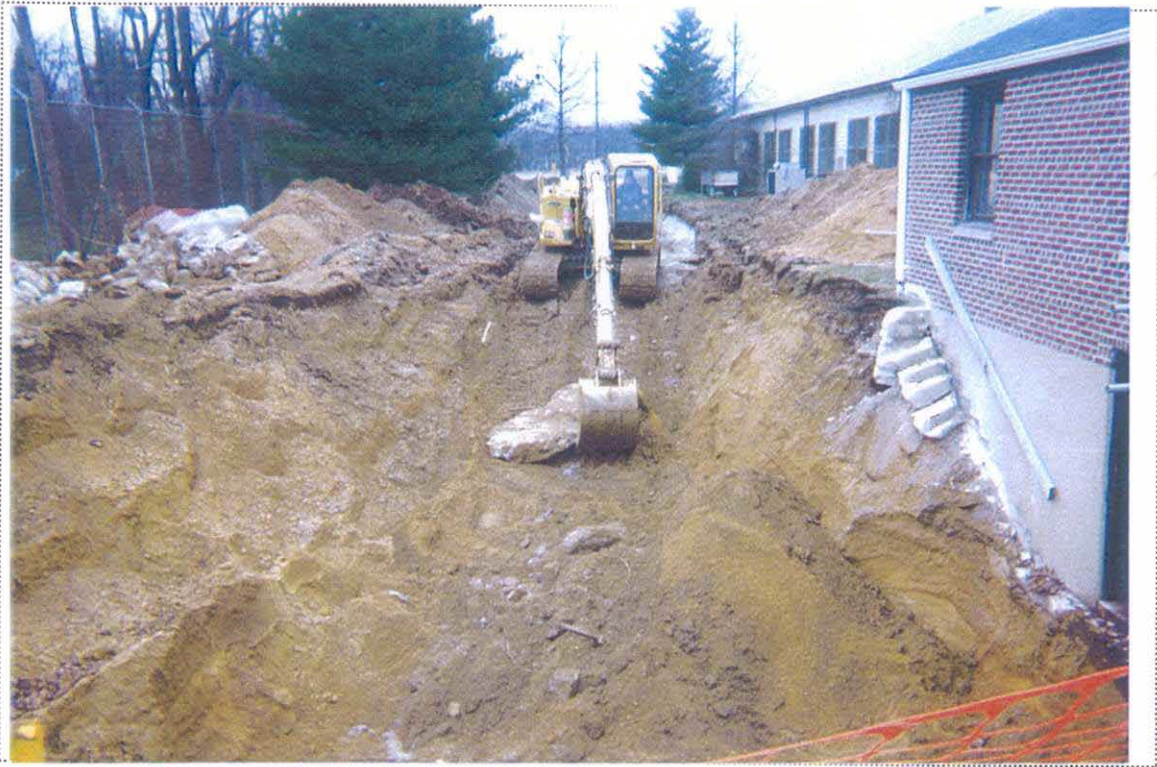
PHOTO 5: View of SMC removing a section of the concrete pad located beneath UST-9064 prior to confirmatory sampling (looking north).
