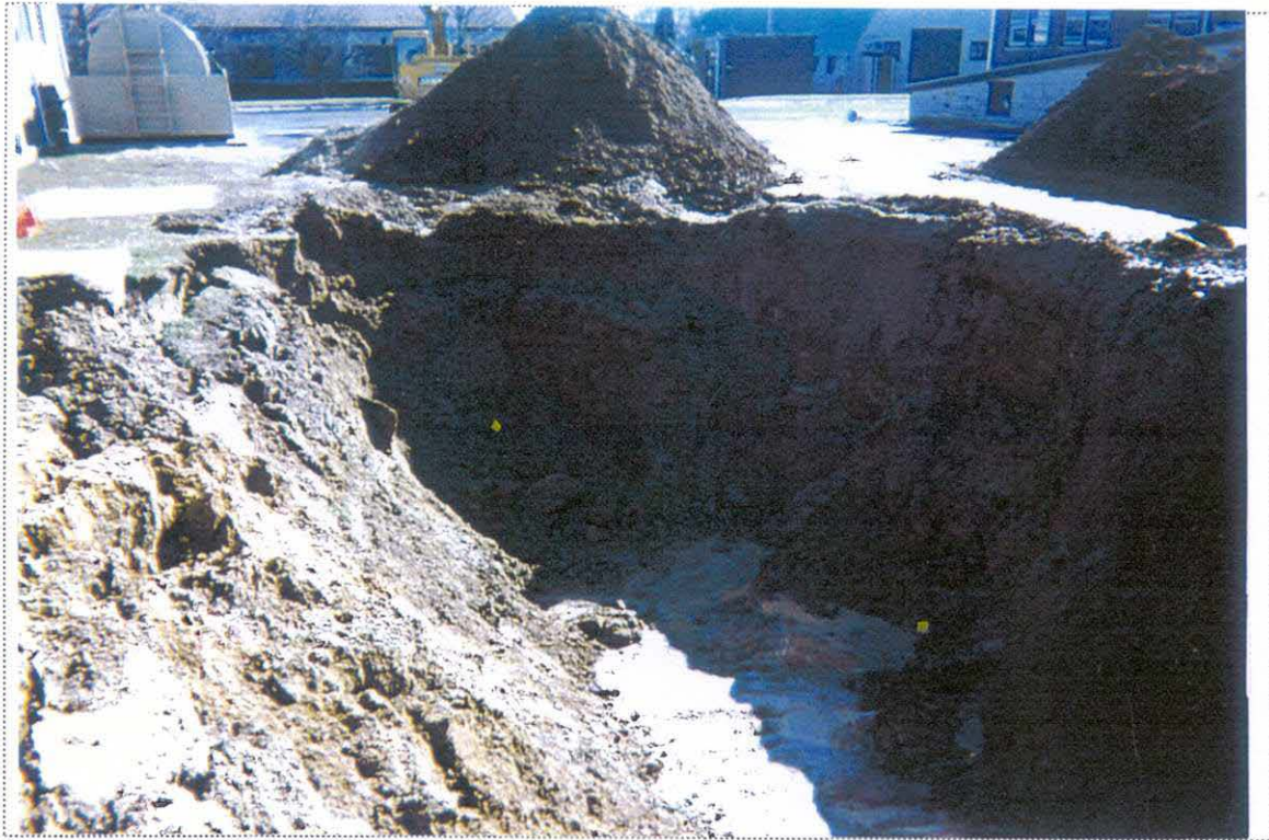
PHOTO 3: View of sampling locations in the UST-9041 excavation (looking south).
