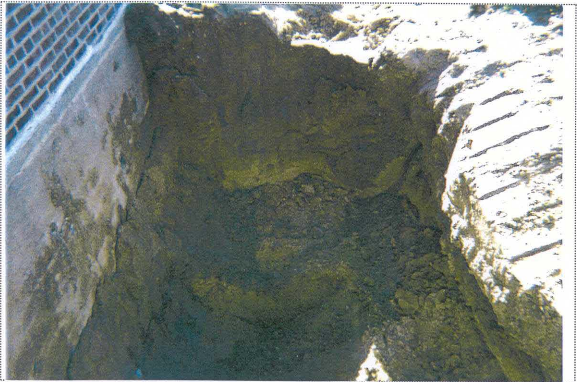
PHOTO 2: View of the UST-9028(B) excavation prior to sampling (looking west).
