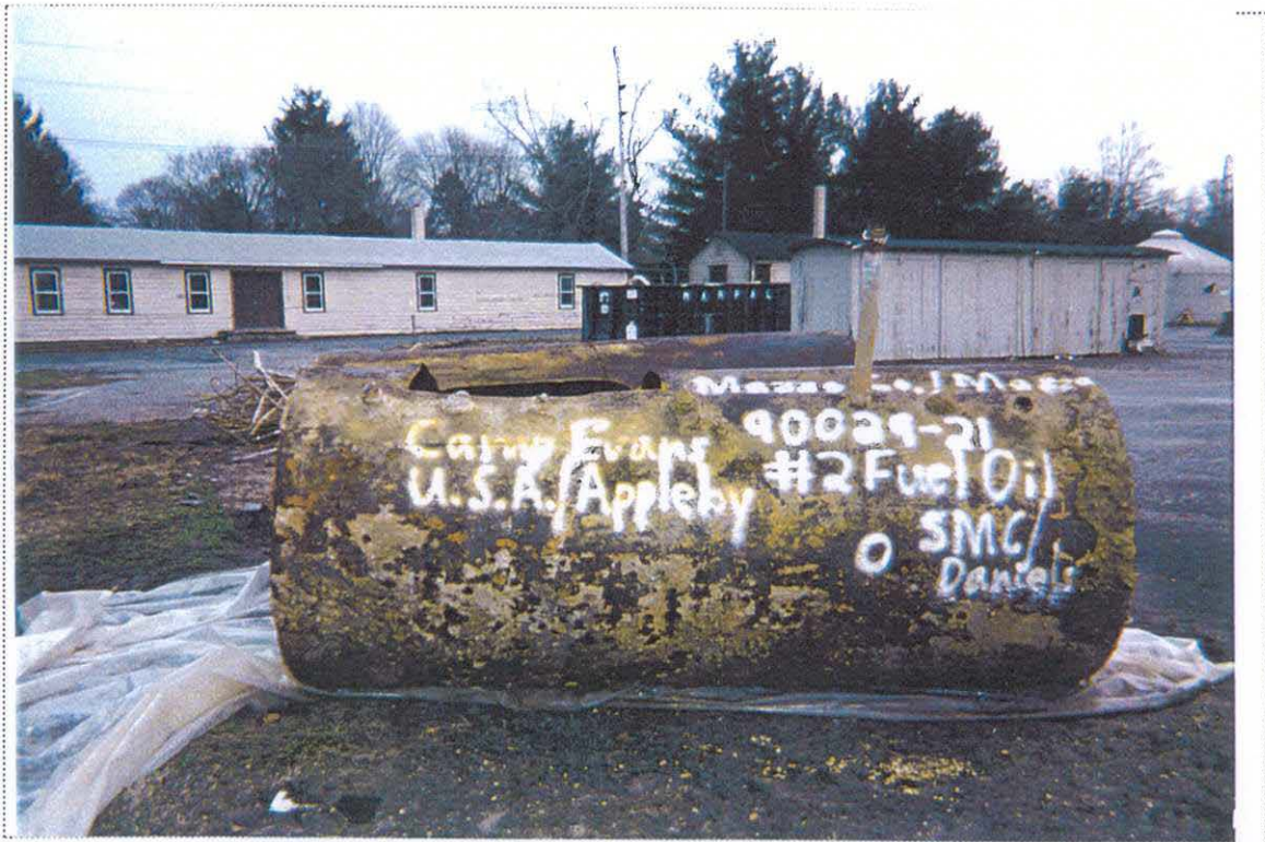
PHOTO 4: View of UST-9051 staged on the west side of Building 9061 awaiting disposal and labeled with all required information.
