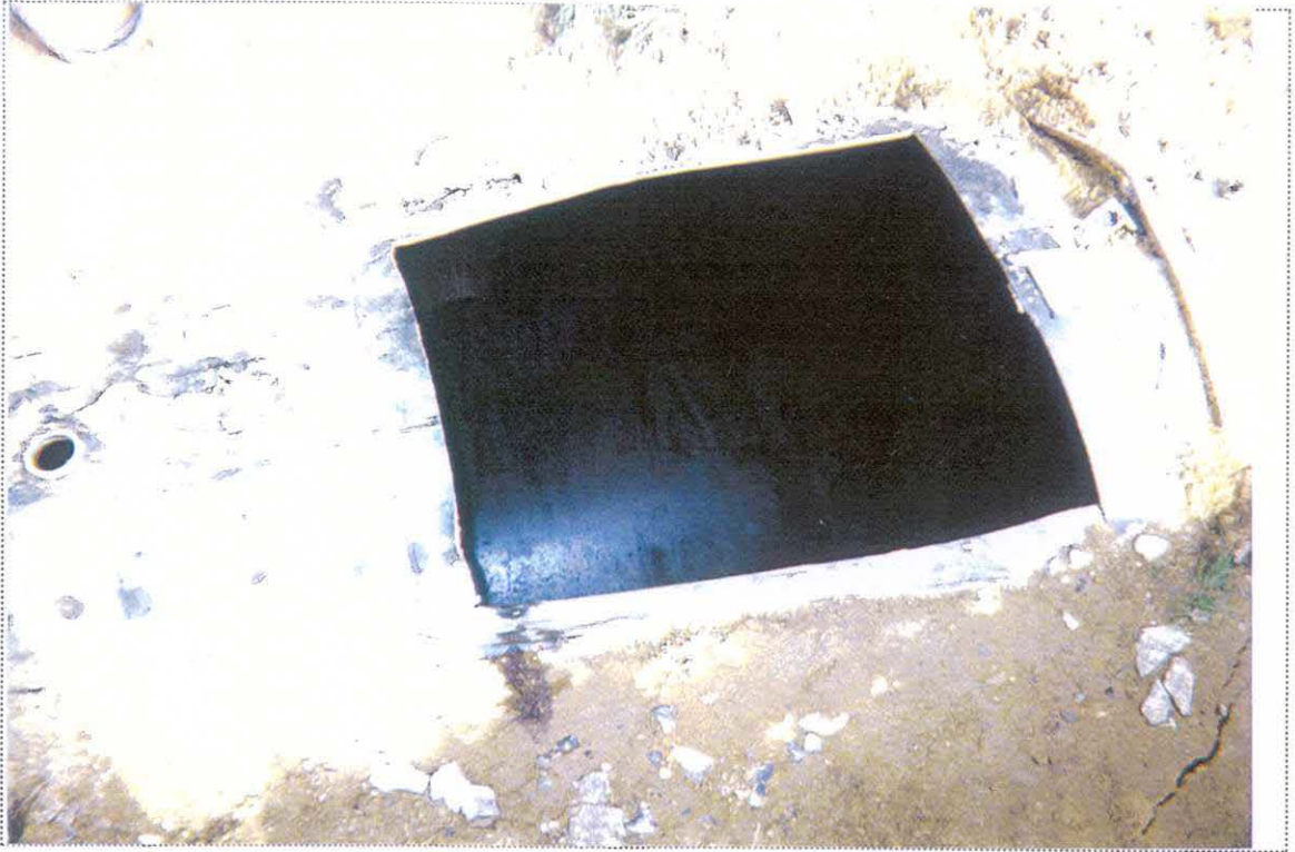
PHOTO 1: View of the cleaned interior of UST-9057(B) (looking east/southeast).
