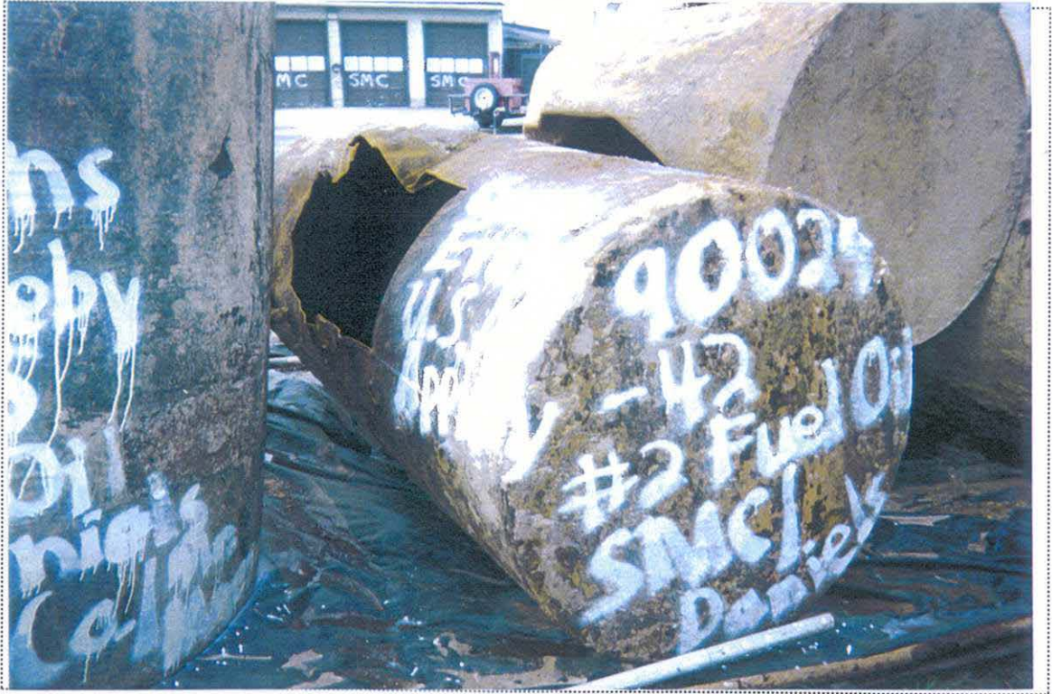
PHOTO 3: View of the UST-9028(B) staged on the west side of UST-9061 awaiting disposal and labeled with all required information.
