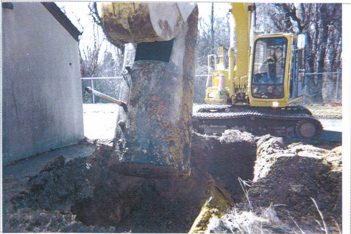
PHOTO 2: View of UST-9051 being removed from the ground (looking west/southwest).
