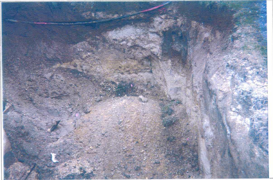
PHOTO 3: View of the sampling locations in the UST-9028(A) excavation (looking east).
