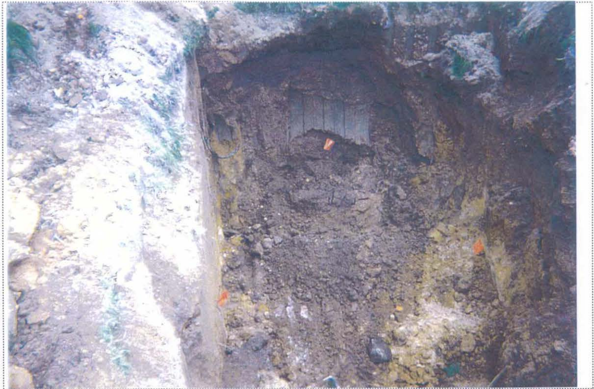
PHOTO 3: View of the sampling locations in the UST-9057(B) excavation (looking north).
