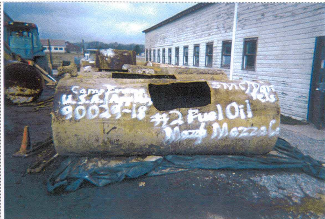
PHOTO 4: View of UST-9045 staged on the west side of Building 9061 awaiting disposal and labeled with all required information.
