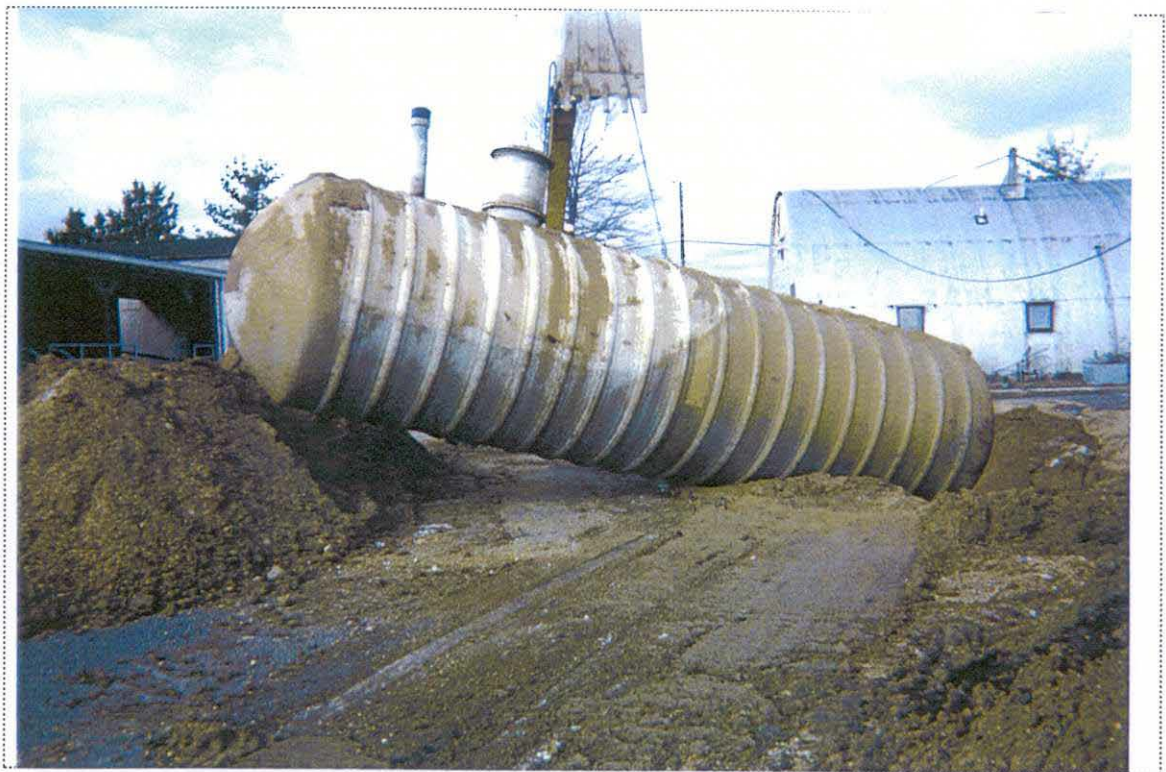
PHOTO 2: View of UST-9041 being removed from the ground (looking north/northwest).
