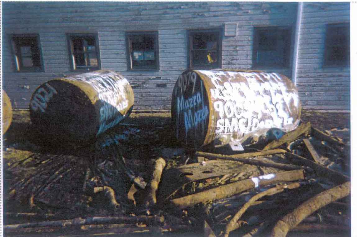
PHOTO 3: View of UST-9079 on the west side of Building 9061 awaiting disposal and labeled with all required information.
