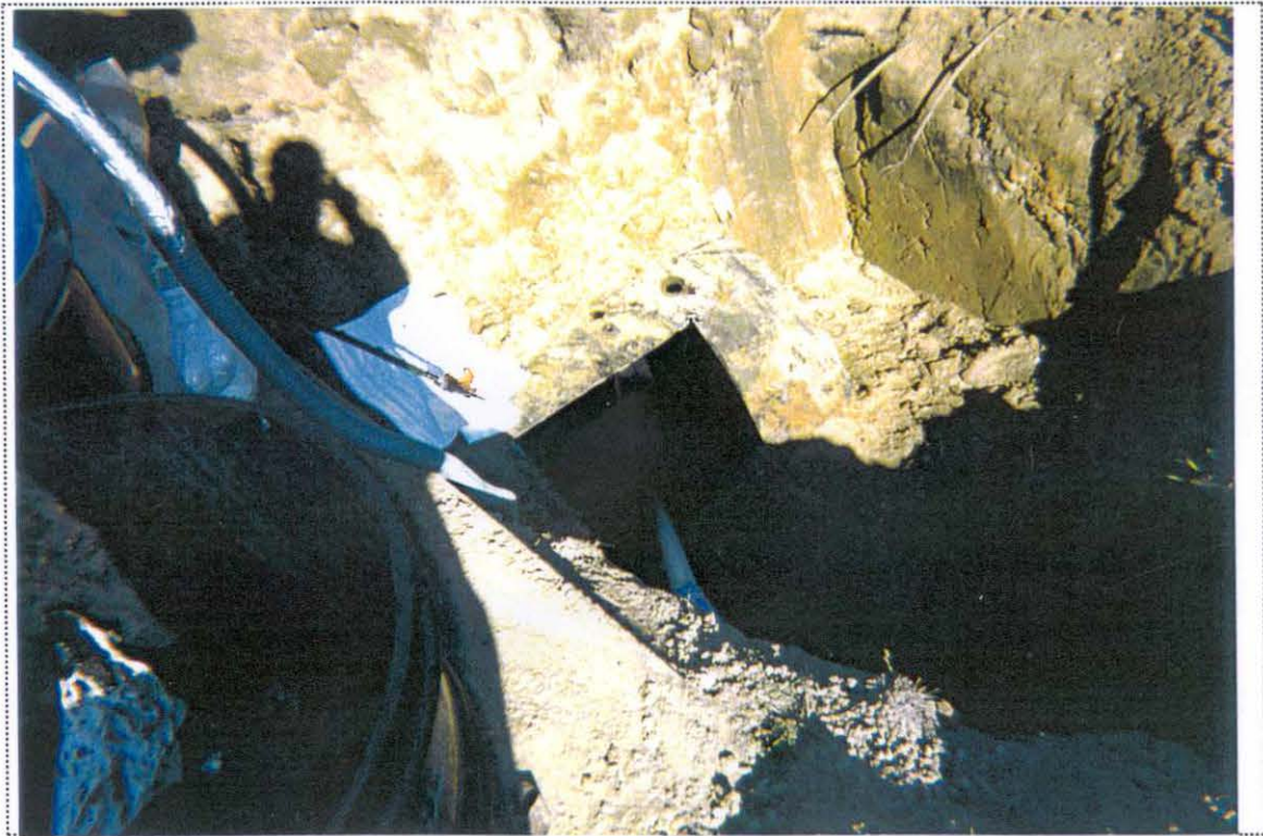
PHOTO 2: View of the cleaning of UST-9028(C) (looking northeast).
