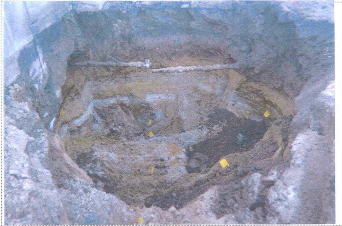
PHOTO 3: View of sampling locations in the UST-9053 excavation (looking west).
