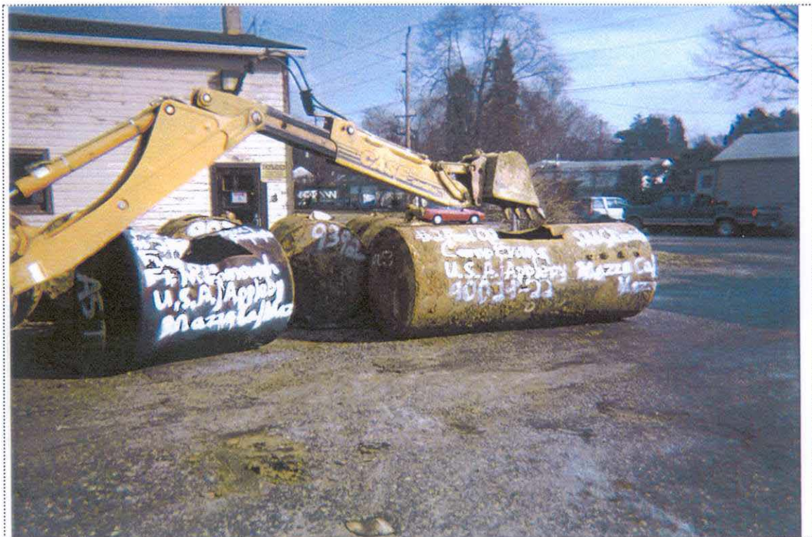
PHOTO 4: View of UST-9053 staged on the west side of Building 9061 awaiting disposal and labeled with all required information.
