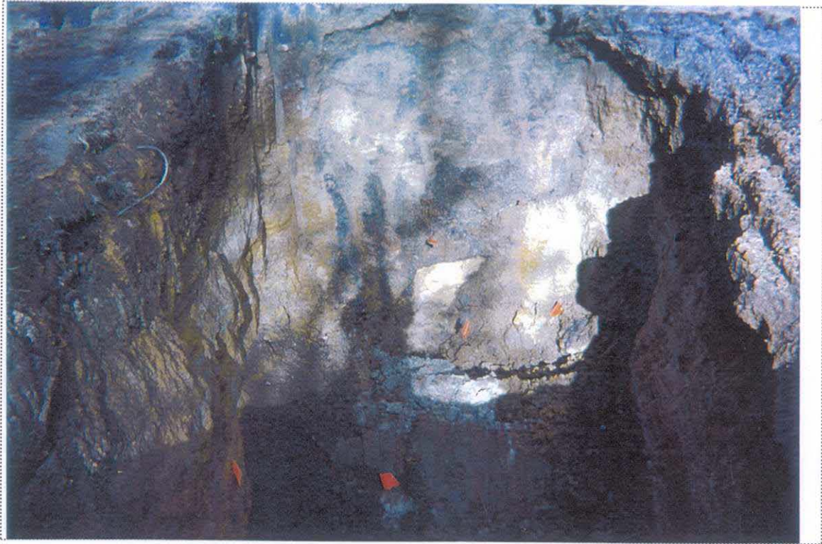
PHOTO 3: View of sampling locations in the UST-9051 excavation (looking east).
