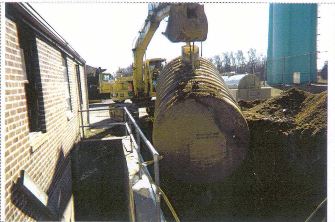
PHOTO 2: View of the UST-9064 being removed from the ground (looking south/southwest).
