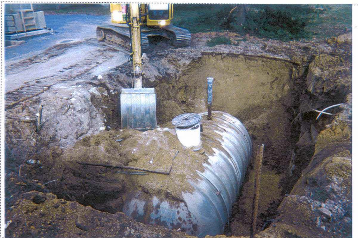
PHOTO 1: View of UST-9033 being uncovered (looking east/northeast).
