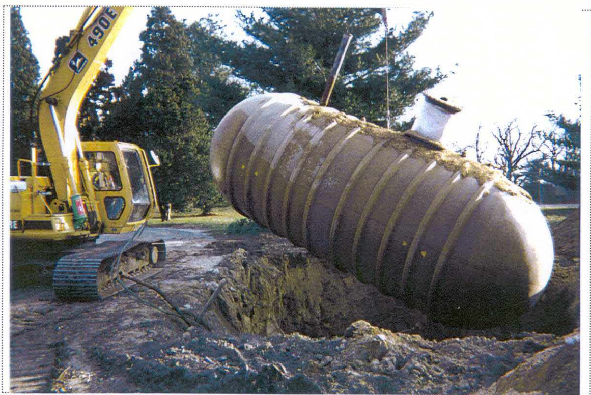
PHOTO 2: View of the UST-9033 being removed from the ground (looking east).
