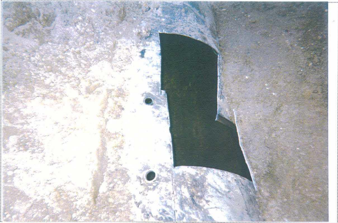
PHOTO 1: View of the cleaned interior of UST-9028(B) (looking east).
