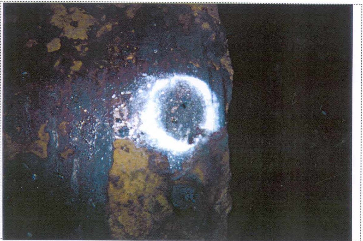
PHOTO 2: View of 0.25 inch hole located at the western end of UST-9053.
