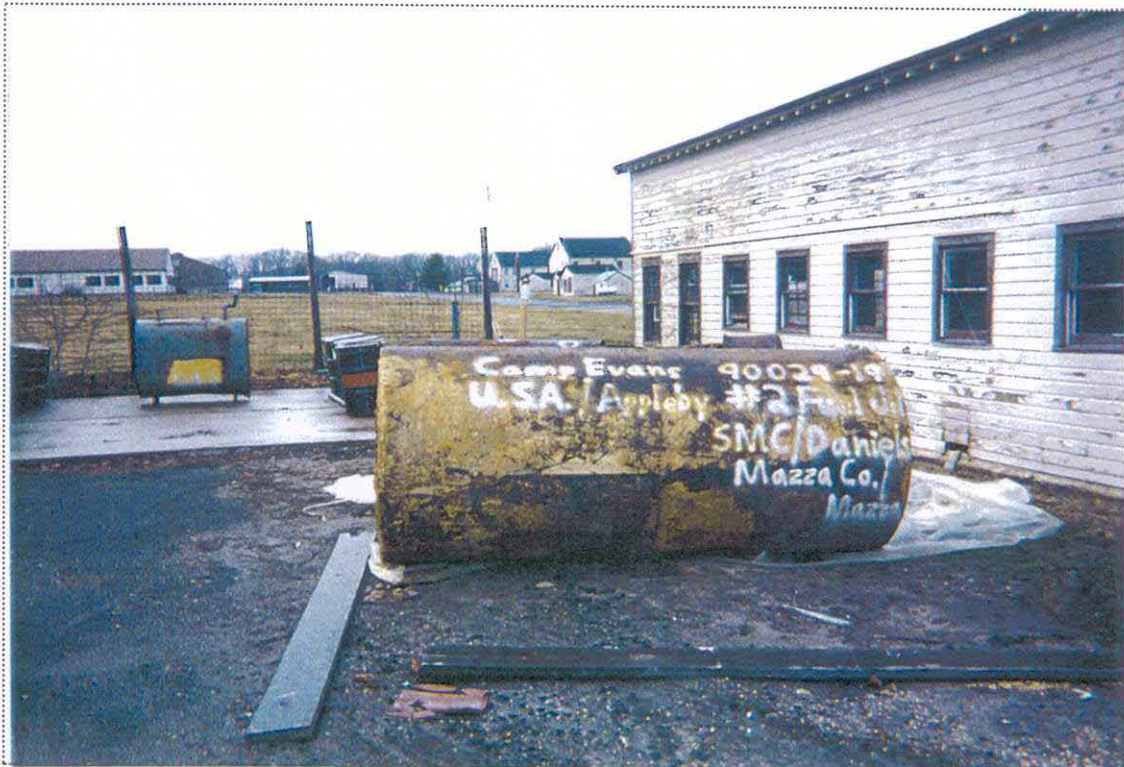
PHOTO 4: View of UST-9047 staged on the west side of Building 9061 awaiting disposal and labeled with all required information.
