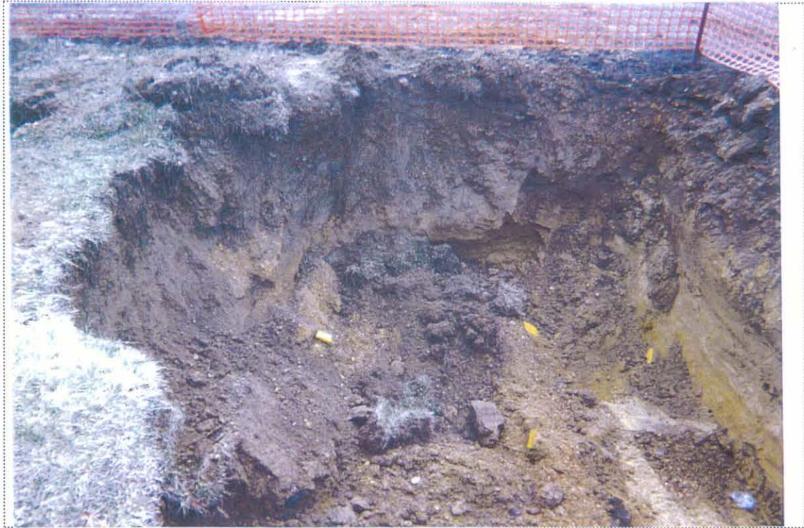
PHOTO 3: View of the sampling locations in the original UST-9055 excavation (looking west).
