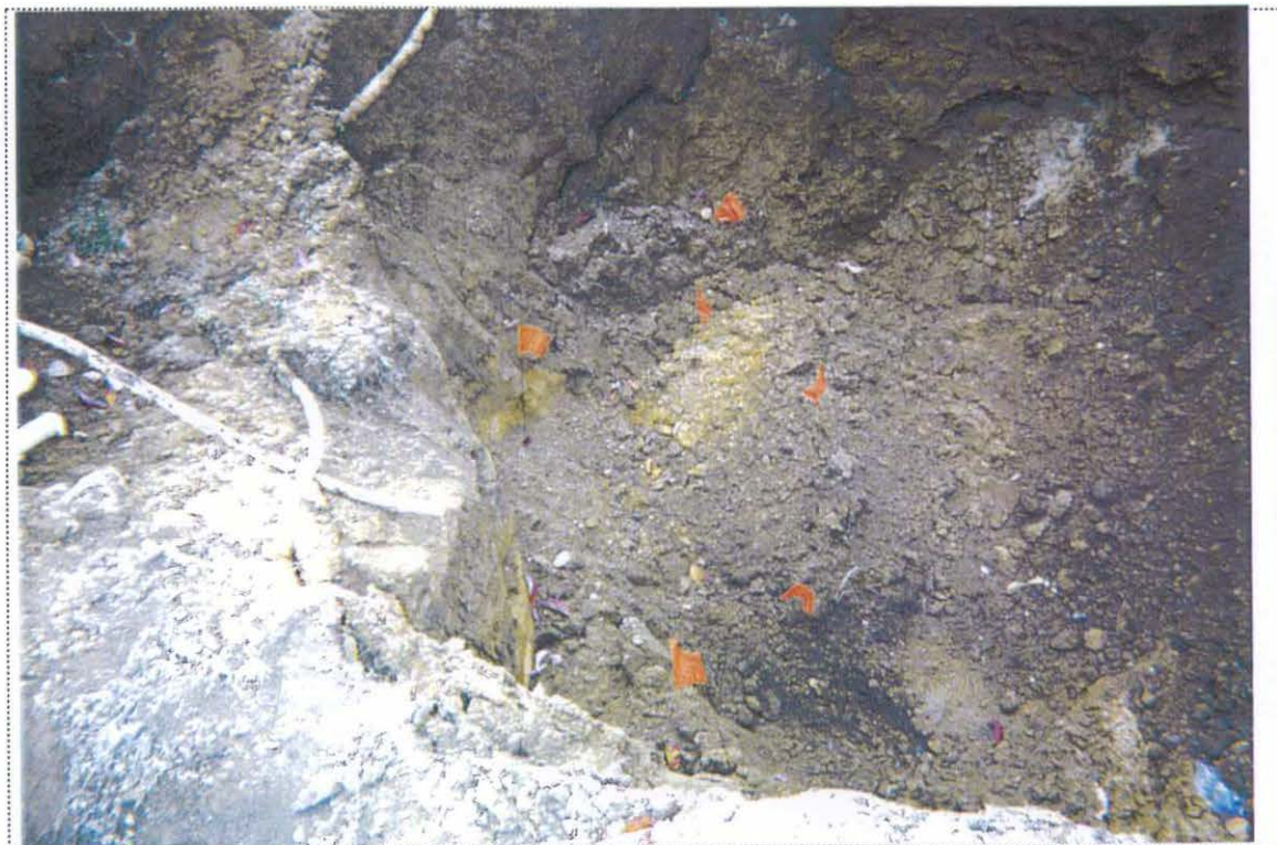
PHOTO 2: View of the sampling locations in the UST-9057(A) excavation (looking north).
