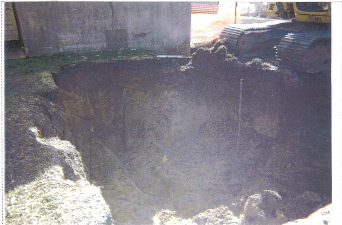
PHOTO 4: View of the sampling locations in the remedial UST-9055 excavation (looking south/southwest).
