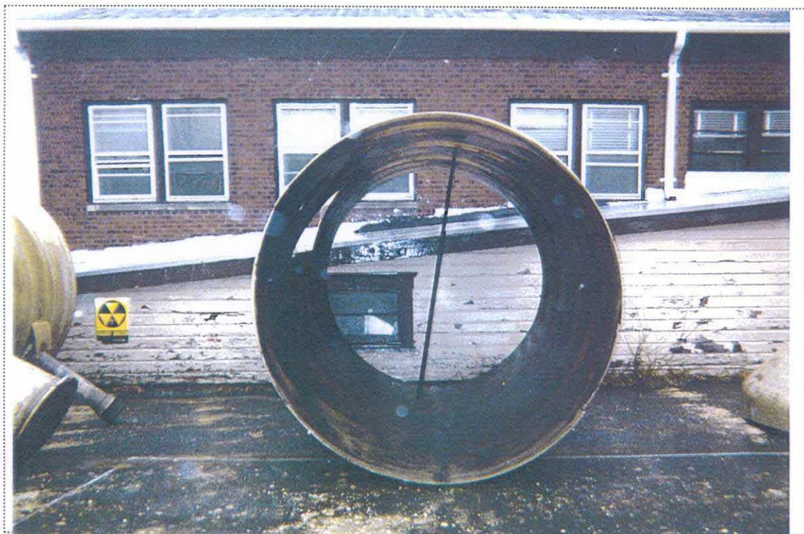
PHOTO 4: View of cleaned sections of UST-9041 awaiting staging in a roll off container for disposal off site.
