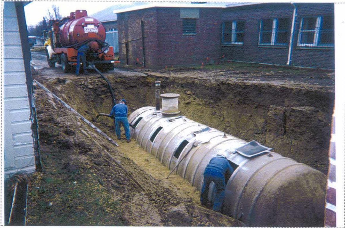
PHOTO 1: View of SMC and Lorco personnel removing oil residue/sludge from the interior of UST-9038 (looking south/southeast).
