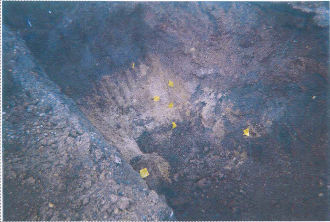
PHOTO 3: View of sampling locations in the UST-9045 excavation (looking north/northeast).
