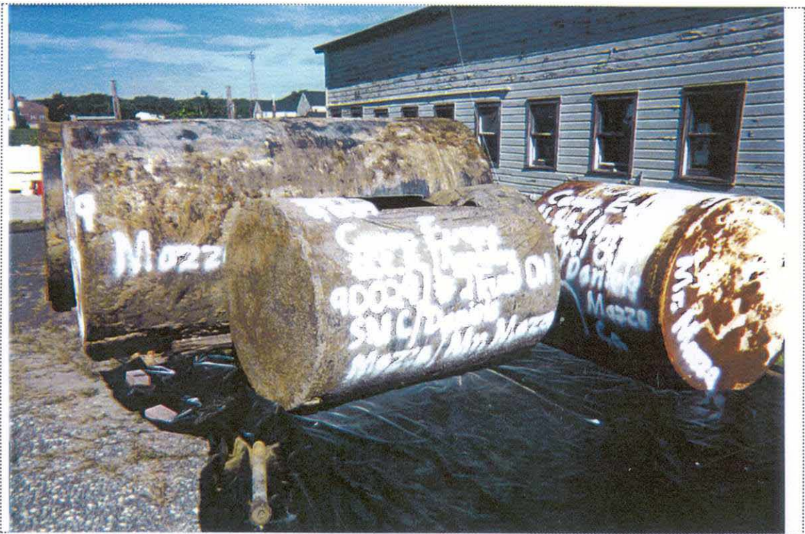
PHOTO 4: View of UST-9059 staged on the west side of Building 9061 awaiting disposal and labeled with all required information.
