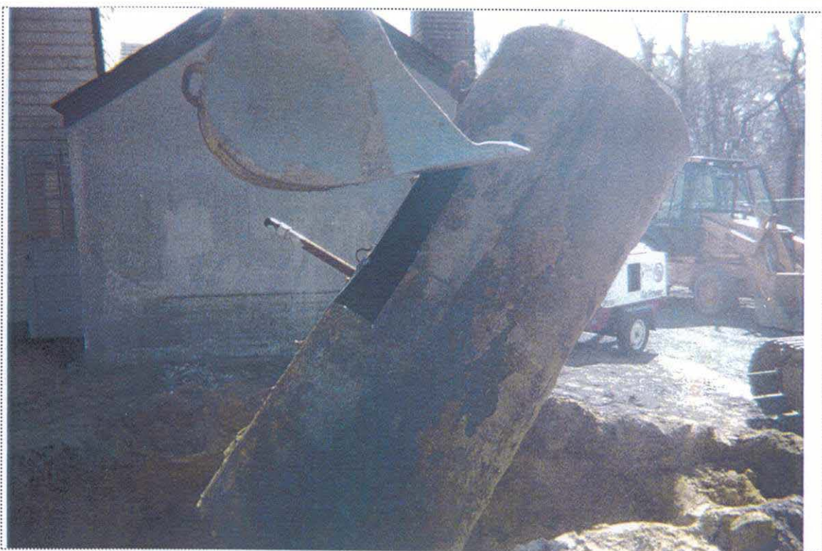
PHOTO 2: View of UST-9047 being removed from the ground (looking south/southwest).
