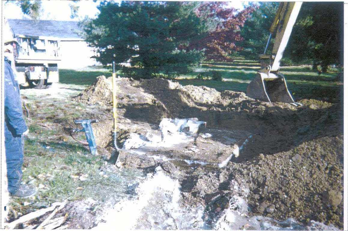
PHOTO 1: View of excavation activities commencing at the UST-9035 location (looking northeast).
