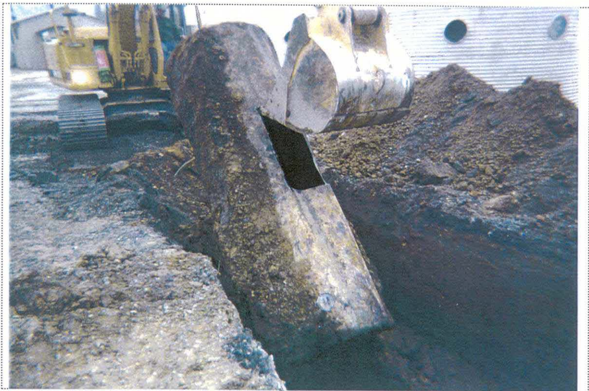
PHOTO 2: View of UST-9045 being removed from the ground (looking south/southwest).
