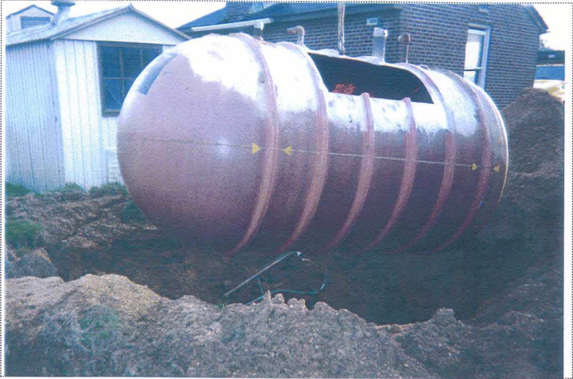
PHOTO 3: View of UST-9030 being removed from the ground (looking southeast).
