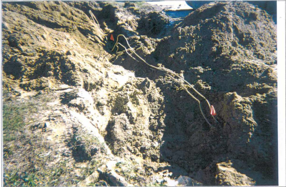
PHOTO 1: View of the sampling locations beneath the return/feed lines (copper tubing) between Building 9028 and UST-9028(C) (looking south/southwest).
