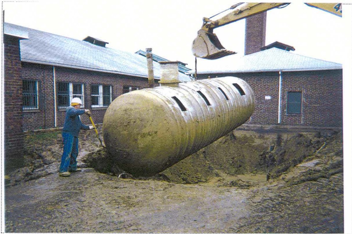
PHOTO 2: View of UST-9038 being removed from the ground (looking northwest).
