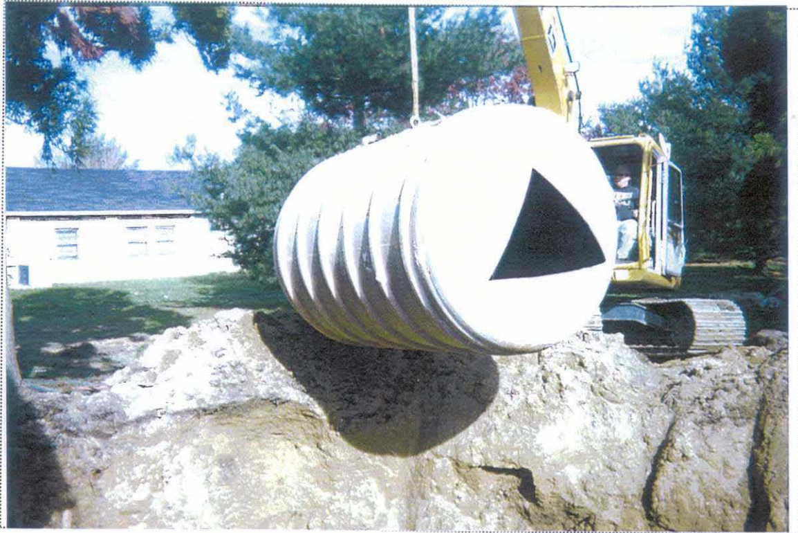
PHOTO 3: View of UST-9035 being removed from the ground (looking northeast).
