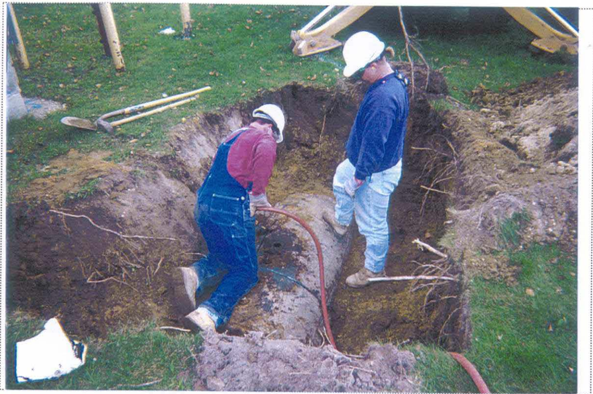
PHOTO 1: View of SMC personnel cutting open the top of UST-9059 (looking south/southeast).
