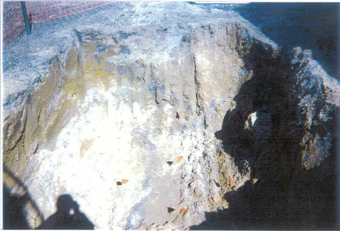
PHOTO 3: View of the sampling locations in the UST-9047 excavation (looking east).
