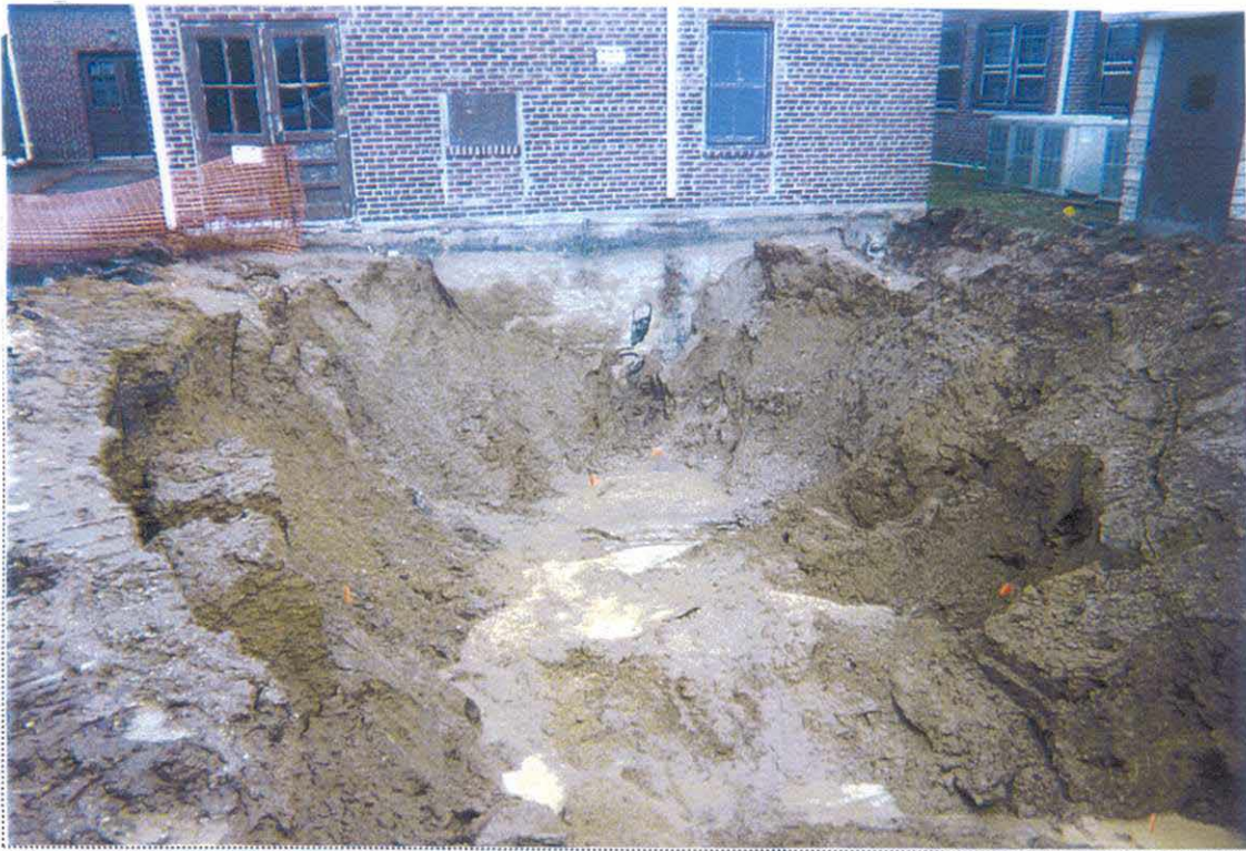
PHOTO 3: View of sampling activities in the UST-9038 excavation.
