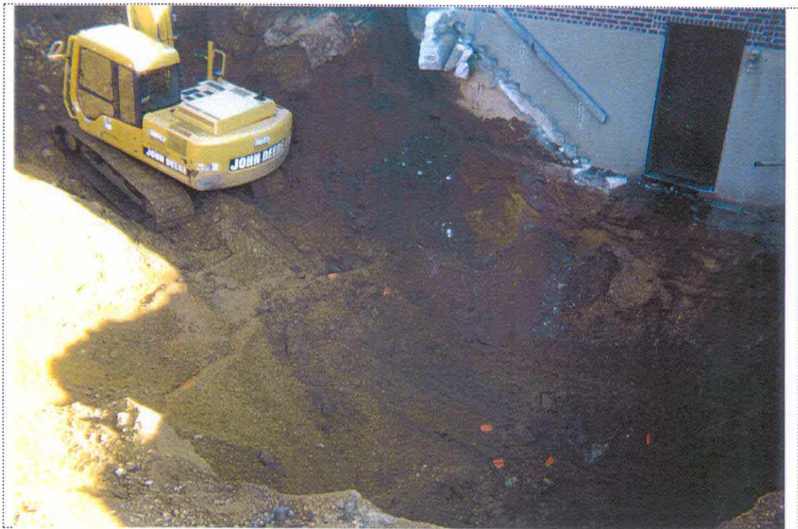
PHOTO 6: View of the confirmatory sampling activities in the UST-9064 excavation (looking northeast).
