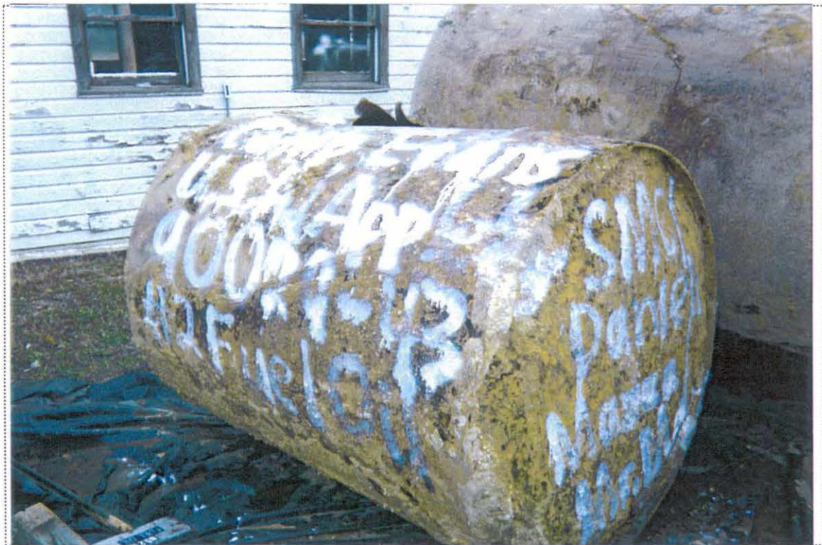
PHOTO 4: View of UST-9028(C) staged on the west side of Building 9061 awaiting disposal and labeled with all required information.
