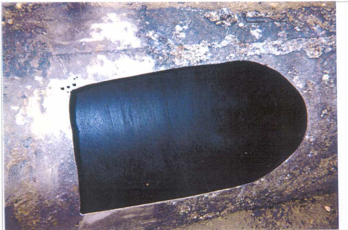
PHOTO 1: View of the cleaned interior of UST-9055 (looking south/southwest).
