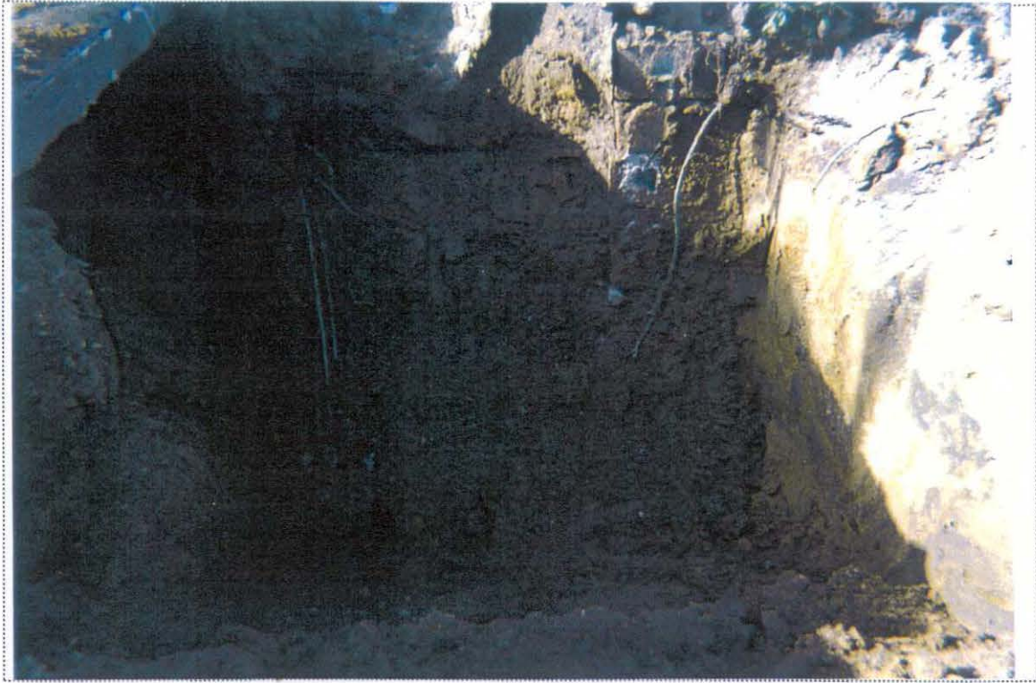
PHOTO 3: View of the UST-9028(C) excavation after removal of the tank (looking north).
