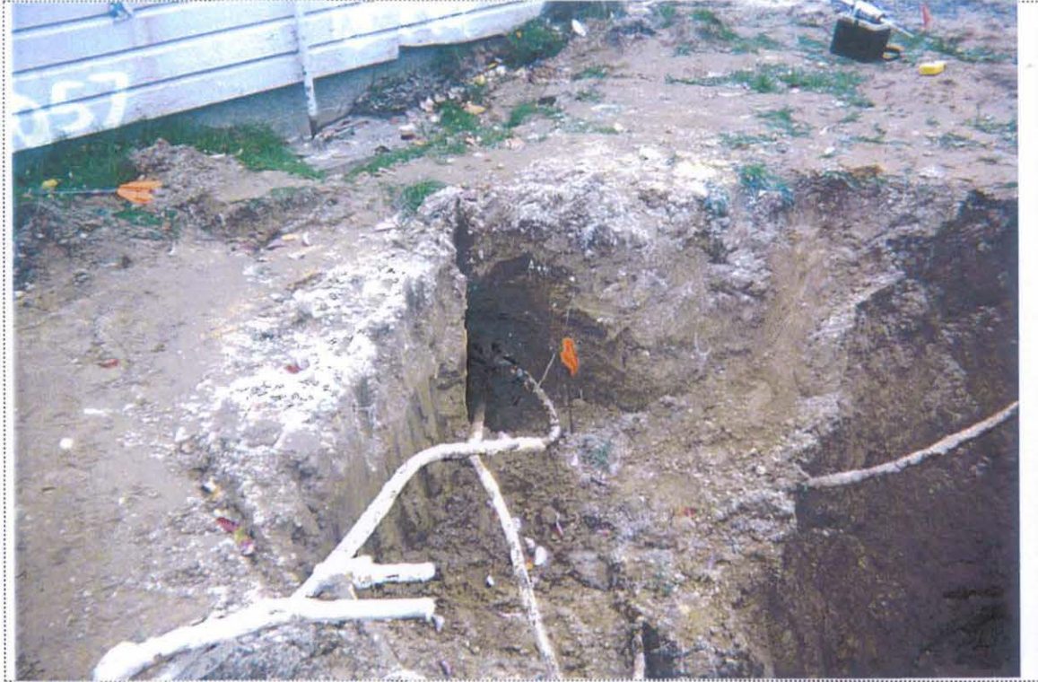
PHOTO 1: View of the sampling location beneath the return/feed line piping of UST-9057(A) (looking northwest).
