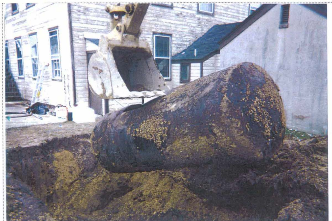
PHOTO 2: View of UST-9055 being removed from the ground (looking southeast).
