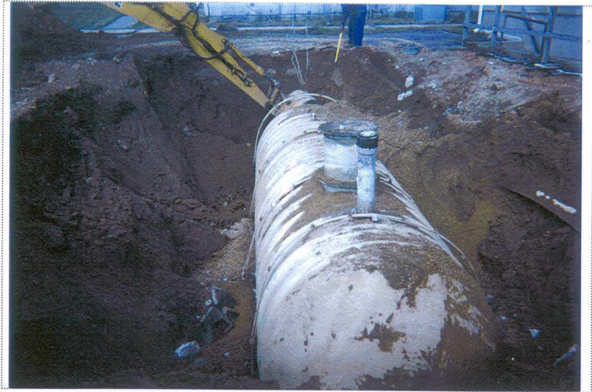
PHOTO 1: View of UST-9041 being uncovered (looking north).
