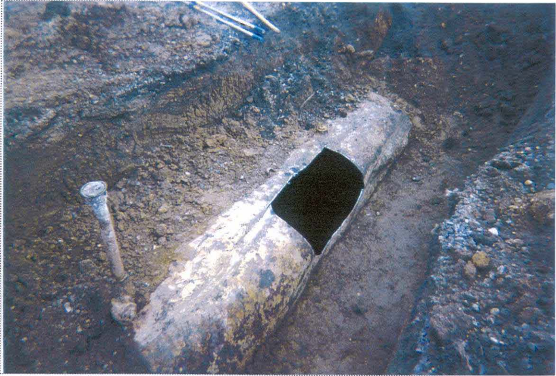
PHOTO 1: View of UST-9045 after cleaning (looking southeast).
