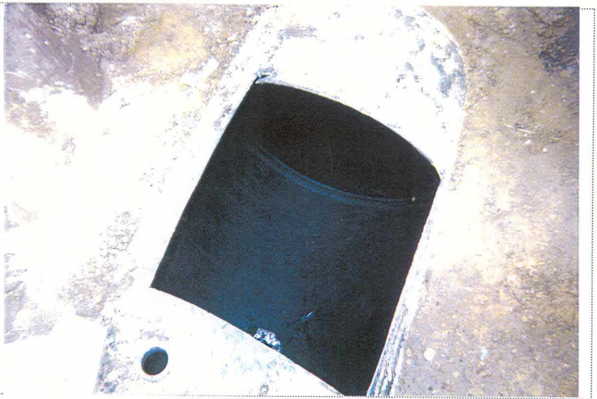
PHOTO 2: View of the cleaned interior of UST-9059 (looking south/southeast).
