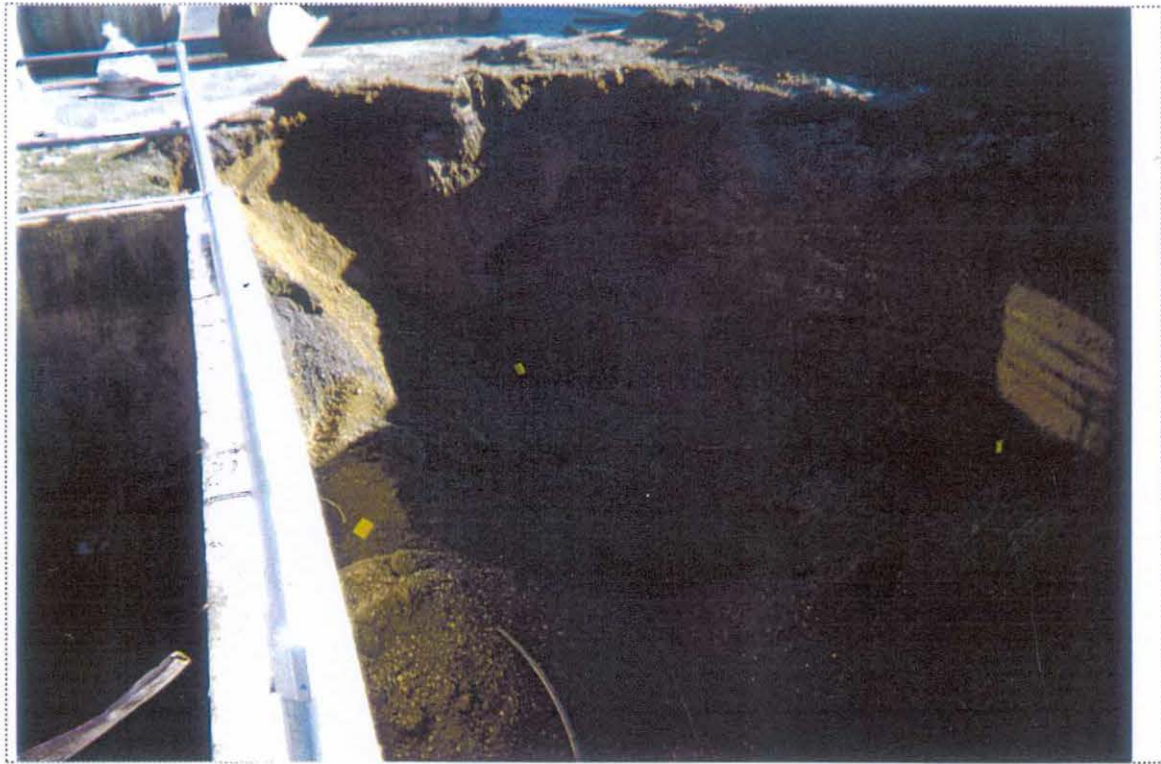
PHOTO 3: View of the sampling locations in the UST-9064 excavation (looking south/southwest).
