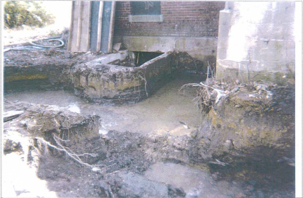
PHOTO 3: View of remedial excavation at Building 9004 to remove contamination caused by a former aboveground storage tank (AST) (looking east/southeast).
