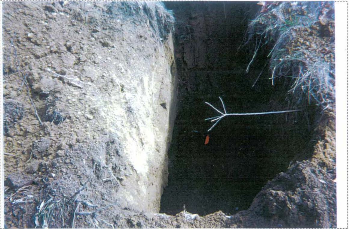
PHOTO 5: View of exploratory test trench adjacent to a former building pad along Watson Avenue (looking south).
