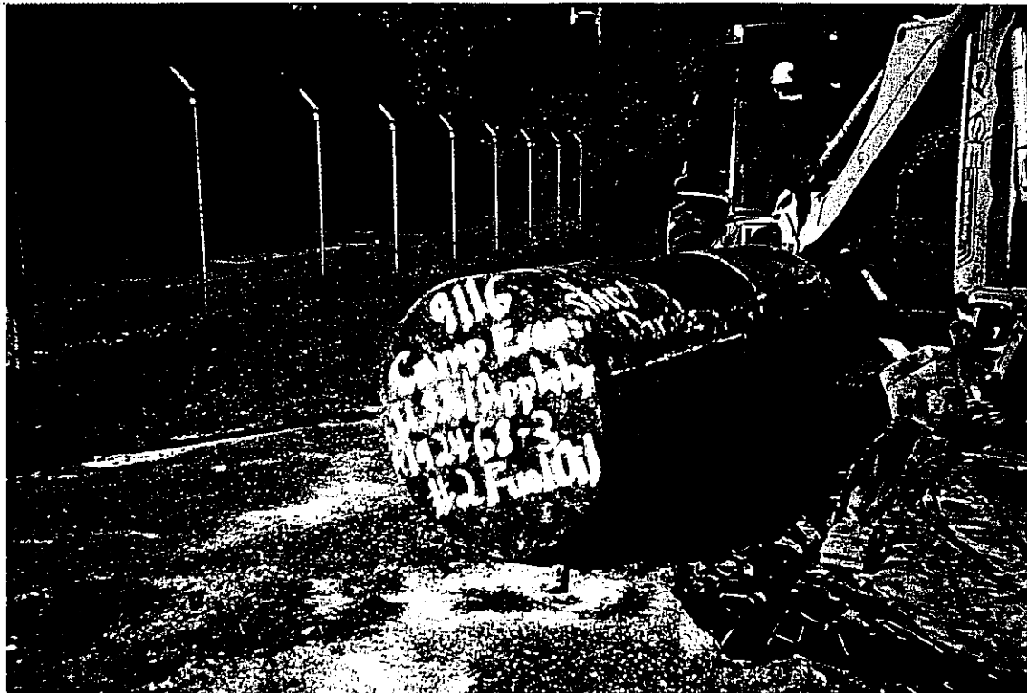
PHOTO 4: View of UST-9116 staged to the south of Building 9062 awaiting removal to Building 9061 (to await permanent disposal) and labeled with all required information.
