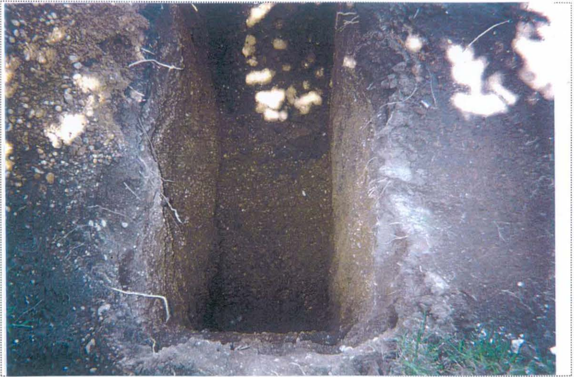
PHOTO 1: View of TP-9043 (Excavation C) where copper tubing with traces of fuel oil/gasoline was found (looking north).
