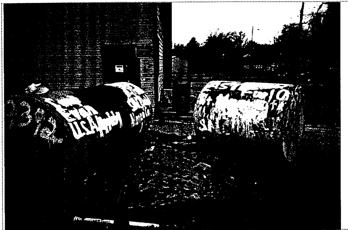
PHOTO 4: View of UST-9392 staged on the west side of Building 9061 awaiting disposal and labeled with all the required information.
