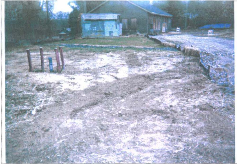
PHOTO 9: View of final site restoration of UST-9007 excavation (looking northeast).
