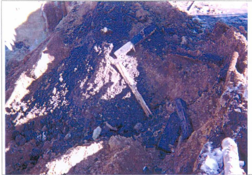
PHOTO 3: View of heavily-stained pieces of former wooden dry well in UST-9007 excavation.
