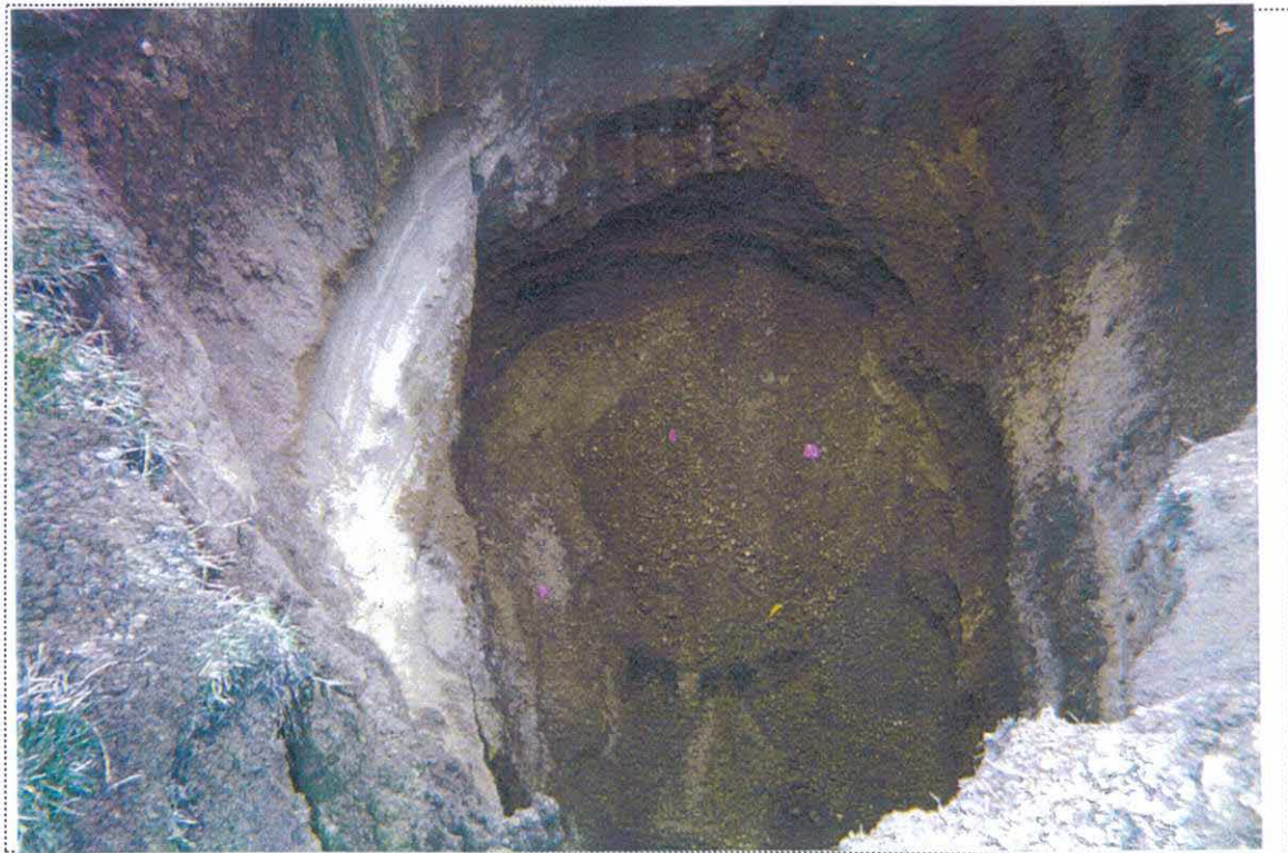
PHOTO 4: View of remedial excavation at Building 9090 to remove contamination caused by a former UST that had been removed previously (looking north).
