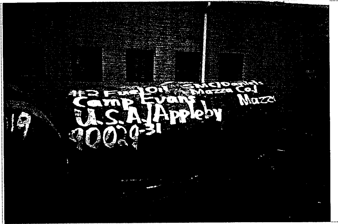
PHOTO 4: View of UST-9100 staged on the west side of Building 9100 awaiting disposal and labeled with all required information.
