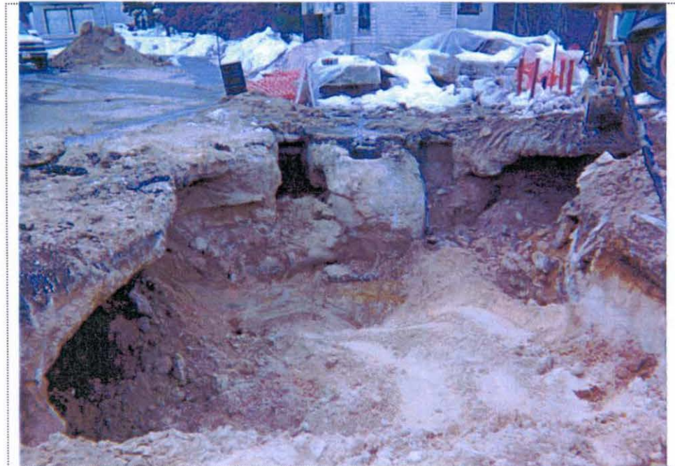
PHOTO 4: View of storm sewer manhole in western end of UST-9007 excavation (looking southwest).
