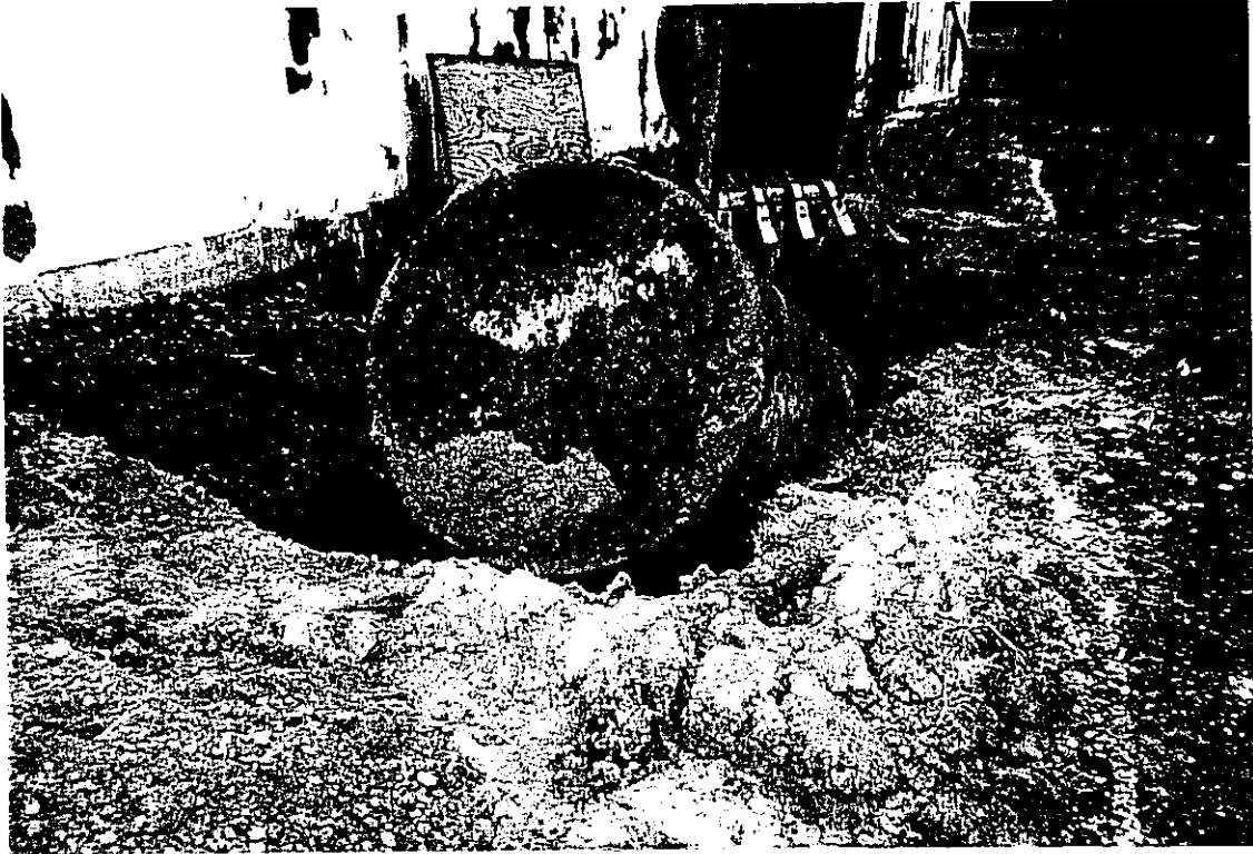
PHOTO 1: View of UST-9307 being removed from the ground (looking south/southwest).
