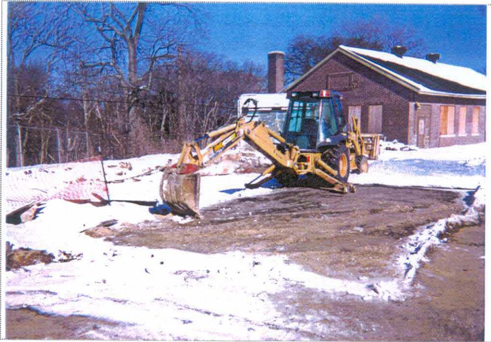
PHOTO 1: View of backhoe beginning UST-9007 excavation (looking northeast).
