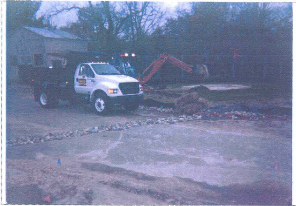
PHOTO 7: View of backhoe beginning to reexcavate storm sewer manhole to remediate PCB contamination in UST-9007 excavation (looking west).
