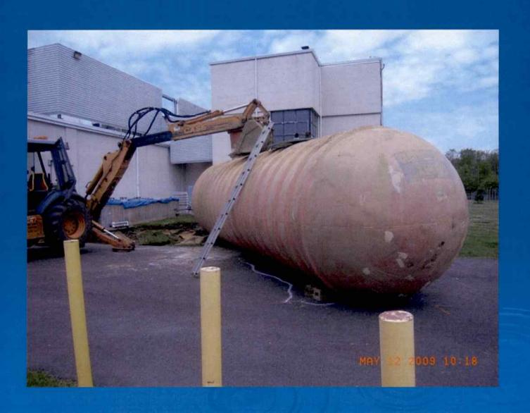
Collect closure samples and backfill excavation with pea gravel and bank run sand.
