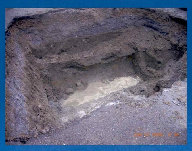
60 cubic yards of petroleum contaminated soil was removed. The excavation was sampled and backfilled.
