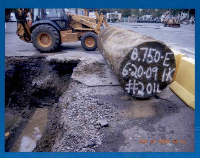
Currently removing contaminated soil from the east and west wall of the excavation.
