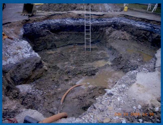
Pumping 300 gallons of fuel and water out of UHOT E.
